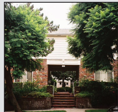
1265 Sweetzer is an example of post-war, multi-family residential apartments.
