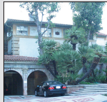
1355 Laurel (Villa d'Este) is an example of an early Courtyard building.
