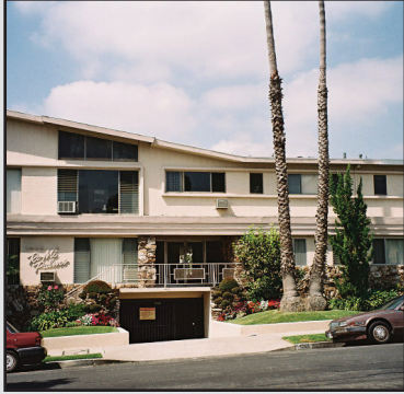
1265 Harper is an example of post-war, multi-family residential apartments.
