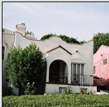
931 Wetherly is an example of the Spanish Colonial Revival style.
