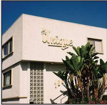
1001 Gardner is an example of the Stucco Box style.
