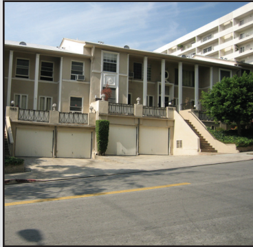
1185 Alta Loma is an example of the Minimal Traditional style.
