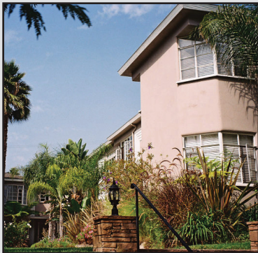
1425 Hayworth is an example of post-war, multi-family residential apartments.
