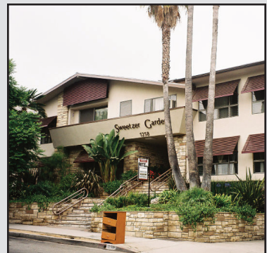
1258 Sweetzer is an example of post-war, multi-family residential apartments.
