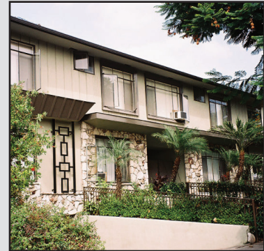
1227 Harper is an example of post-war, multi-family residential apartments.
