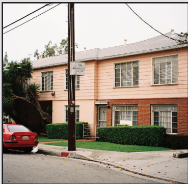
1009 Sweetzer is an example of post-war, multi-family residential apartments.
