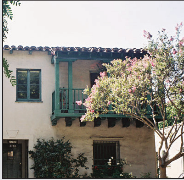
1153 Vista is an example of the Spanish Colonial Revival style.
