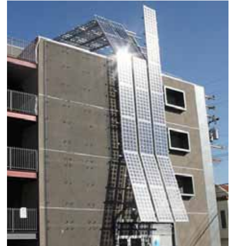
The Sierra Bonita Apartments feature solar collectors on the roof and west façade.
