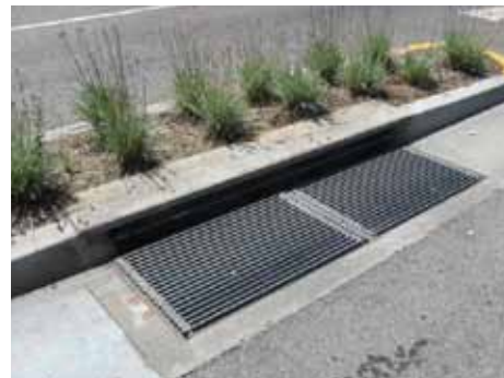
New catch basins were installed as part of the Santa Monica Boulevard Reconstruction Project.
