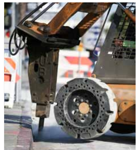
The City's ongoing improvements to roads have resulted in good conditions citywide.
