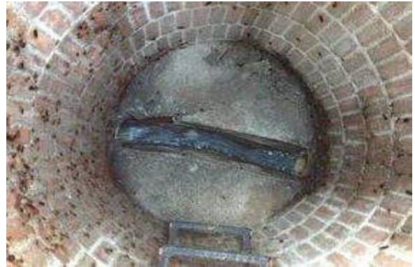
Manhole Before Install
