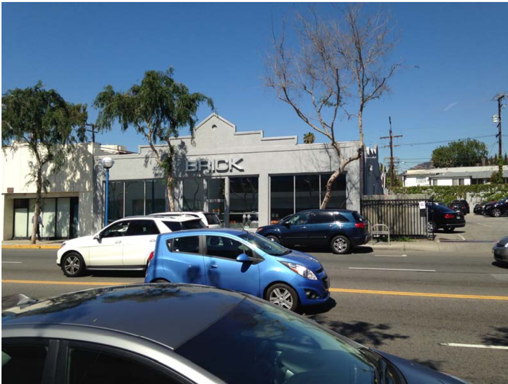
View of the front (south) side of the subject property building 7811 Santa Monica Blvd, West Hollywood
