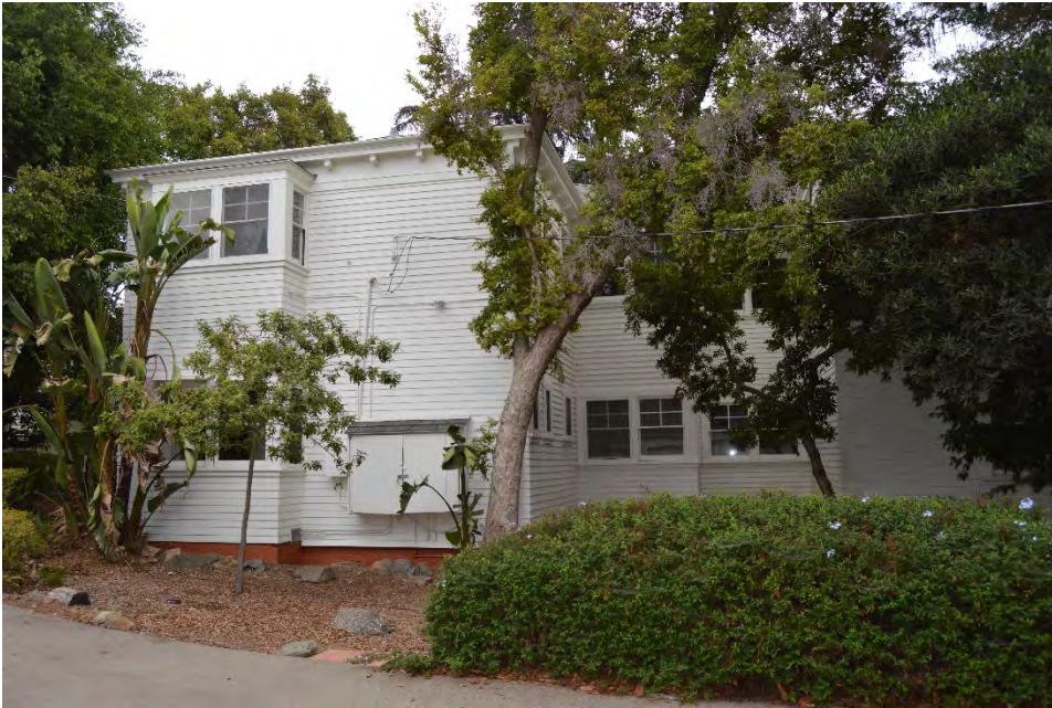
Main Residence; west façade. View to the east.
