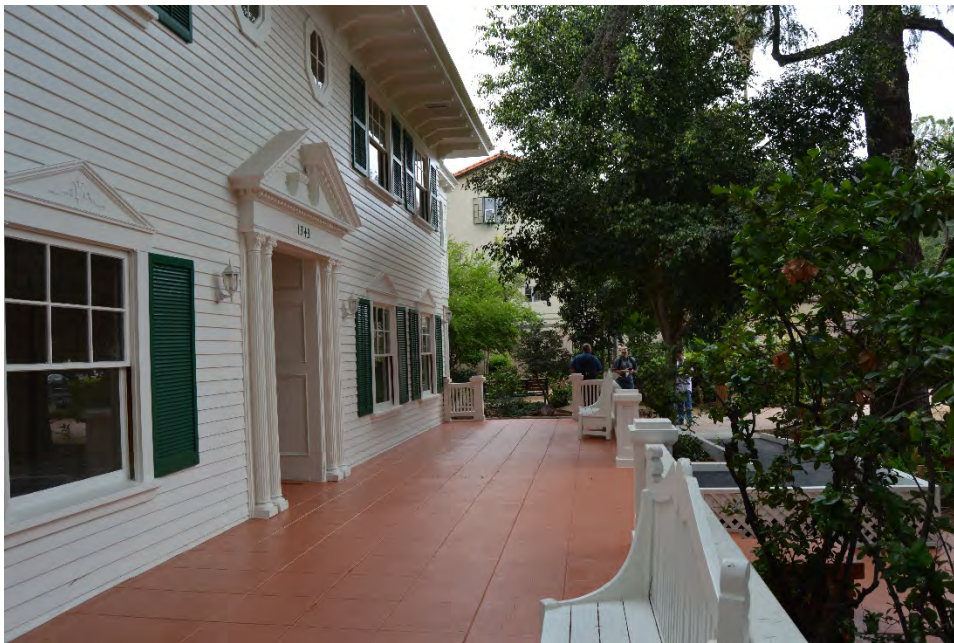
Main Residence; east (primary) façade front porch. View to the east.
