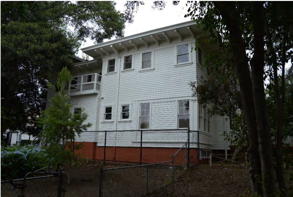
Main Residence; south façade. View to the northwest.
