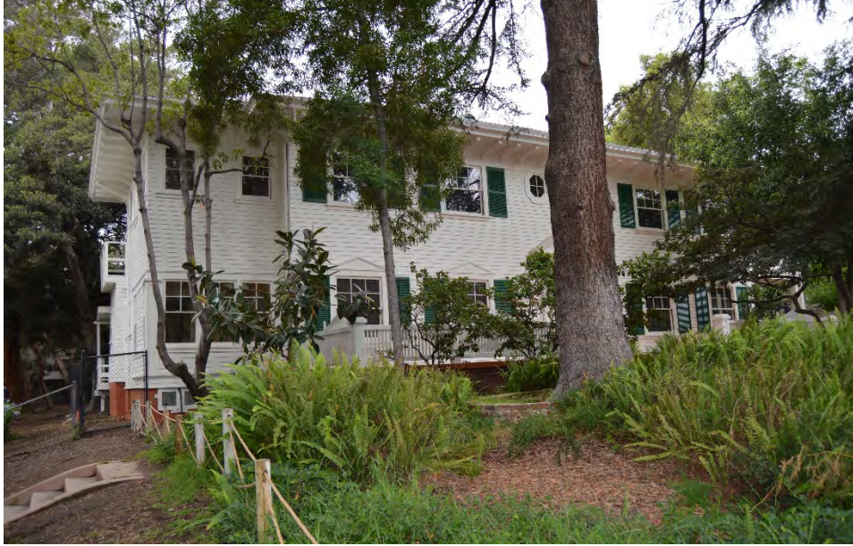
Main Residence; east (primary) façade. View to the northwest.
