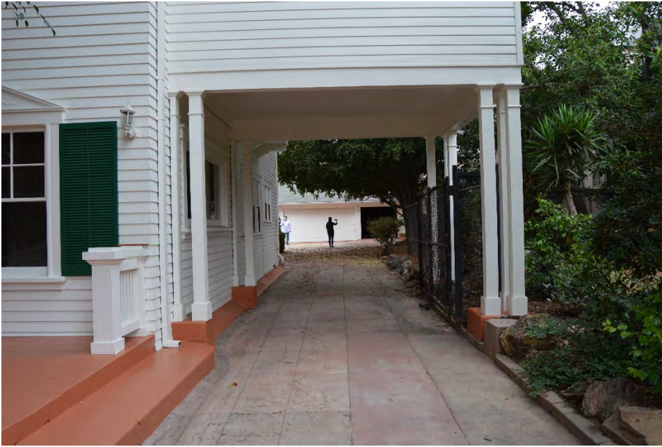
Main Residence; east (primary) façade with driveway and porte cochere. View to the west.
