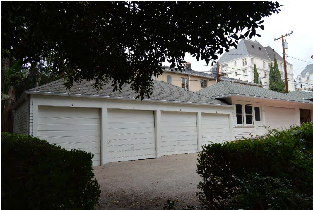
South Garage; east façade. View to the northwest.
