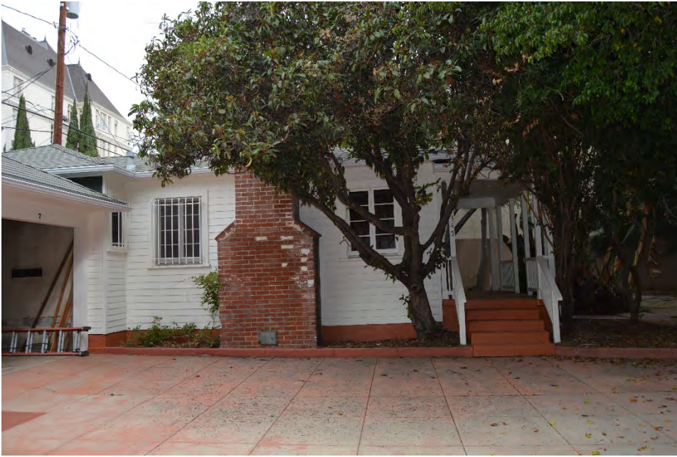
Chauffer's Cottage; south façade. View to the north.
