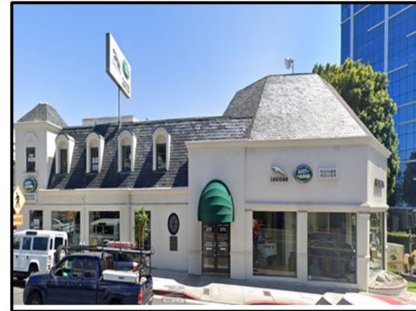
PHOTO 2: View of the northern portion of the project site with a car dealership.
