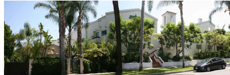
4. W KNOLL DRIVE LOOKING SOUTH
