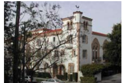
High-density residential buildings use variations in height and massing to enhance existing neighborhoods.
