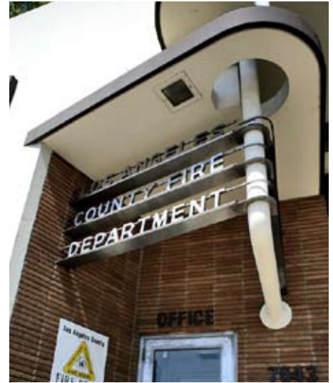
Los Angeles County Fire Station #8 on Santa Monica Boulevard.
