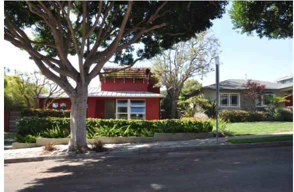
☑ Use of sloped roof forms and lower plate heights reduces the perceived scale of this two-story building.
