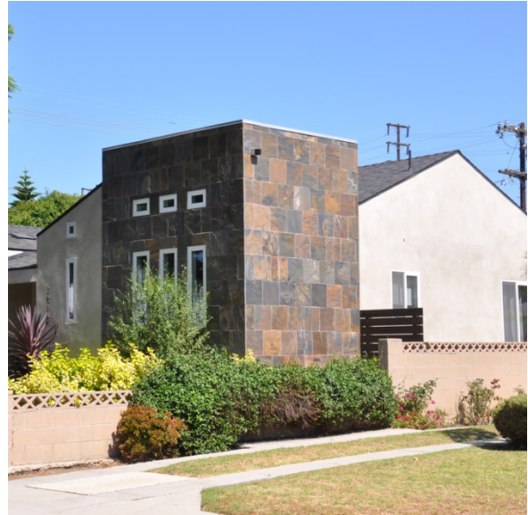
⊗ Addition is out of scale and appears mismatched to original building.
