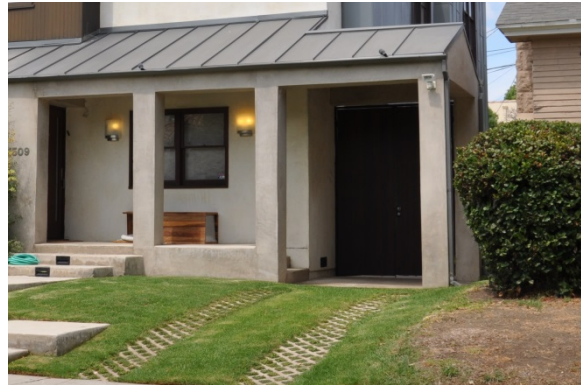
☑ A simple geometric paving system integrates the driveway into the landscape.
