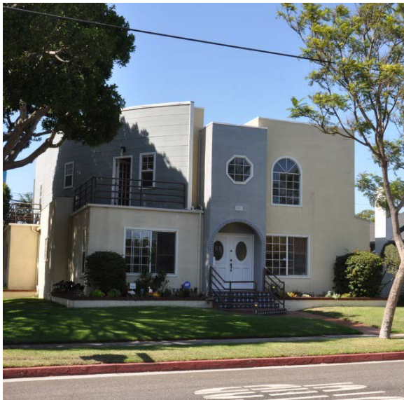
⊗ This building mixes window and door shapes in an inconsistent manner.
