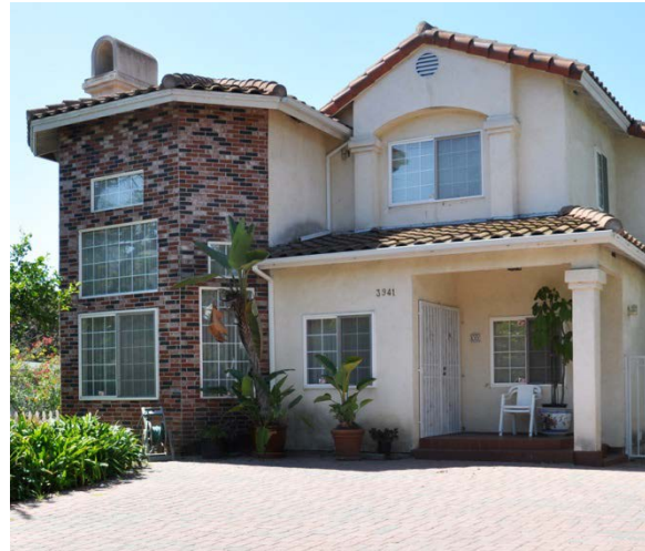
⊗ The transition between brick and stucco is poorly conceived, creating an unintegrated and unfinished appearance.
