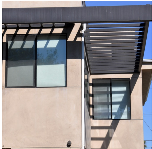
☑ Visual interest, shade and shadow are provided by this architectural feature.
