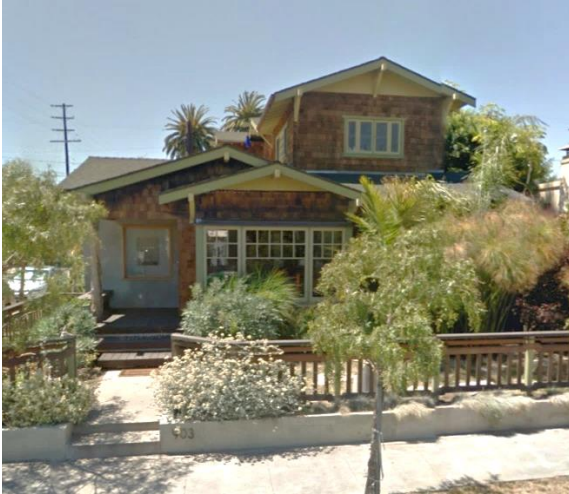
☑ This second-story addition is unified with the original one-story bungalow through a consistent design concept.
