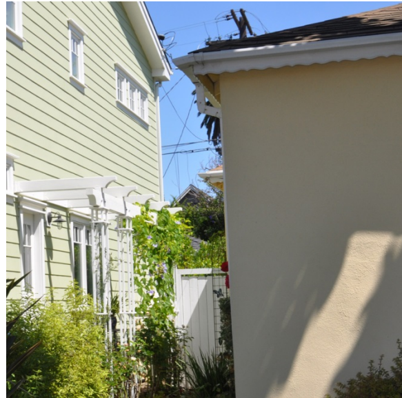
☑ Small side windows at the second story along with trellis at the first floor balance the needs of light and privacy.
