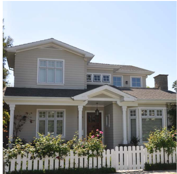
☑ The window proportions are appropriate for this revival style home.
