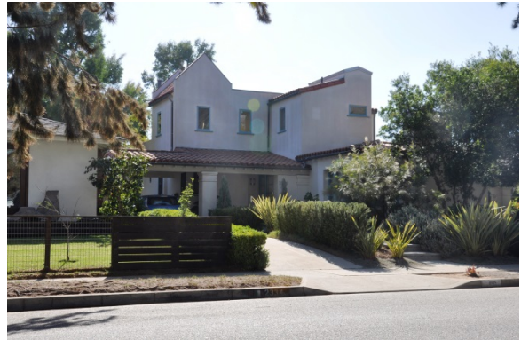
⊗ Use of multiple roof slopes and small gable forms make this home disproportionate to others in the neighborhood.
