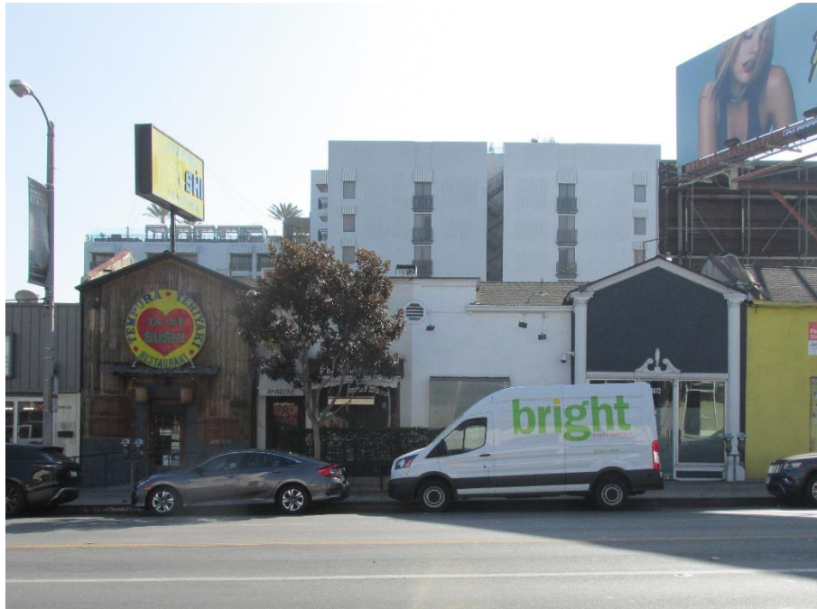
Figure 1. 8866-8872 Sunset Boulevard North Elevation, View looking south (IMG_8995)
