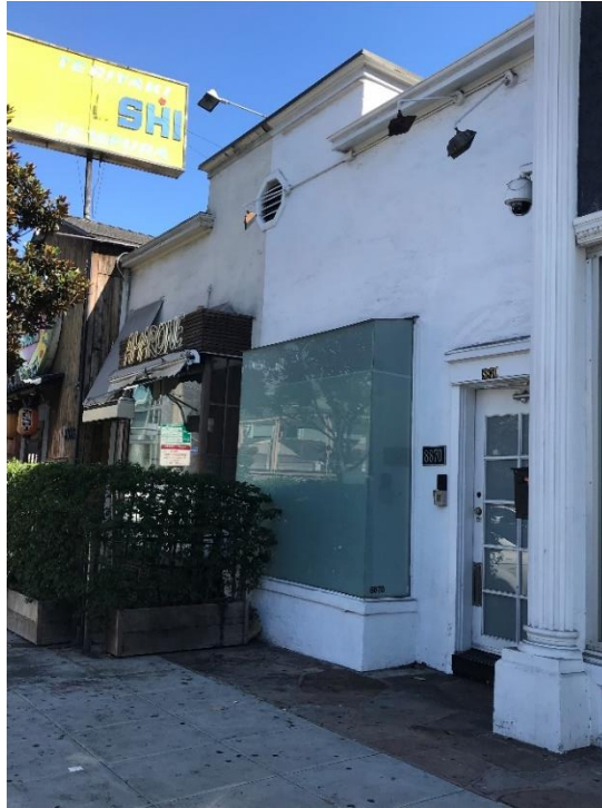
Figure 4. Storefront 2, 8870 Sunset Boulevard (Amarone), North Elevation, View looking southeast (IMG_1497)
