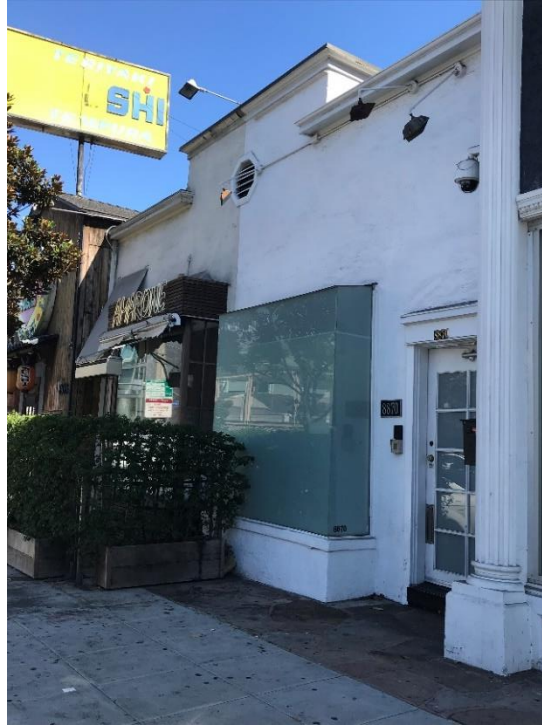
Figure 26. Storefront 2, 8868 Sunset Boulevard (Amarone), North Elevation, View looking southeast (IMG_1497)
