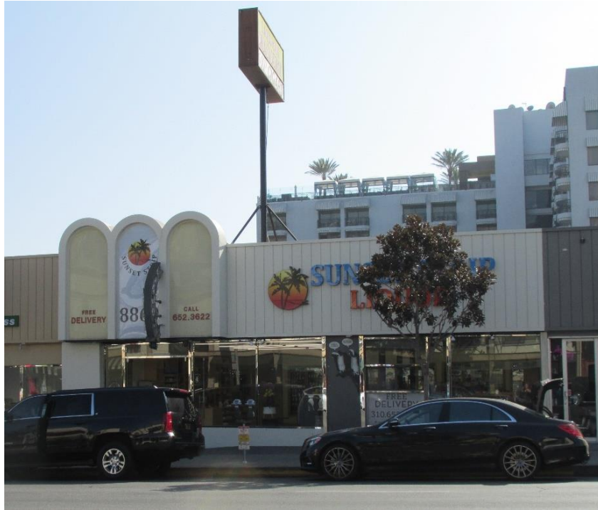
Figure 21. Storefront 2, 8860 Sunset Boulevard (Sunset Strip Liquor) North Elevation, View looking south (IMG_8987)
