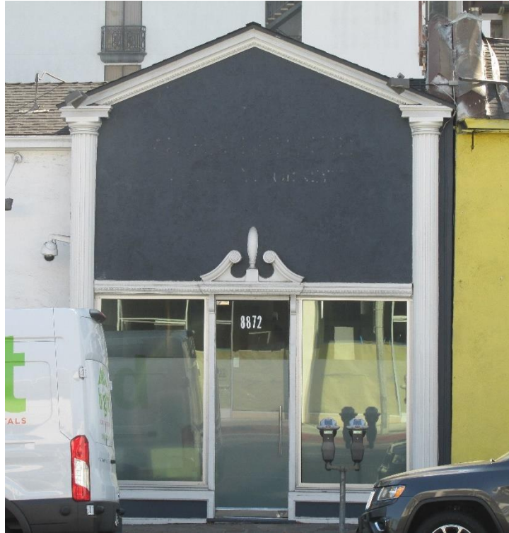
Figure 27. 8872 Sunset Boulevard North Elevation, View looking south (IMG_8998)
