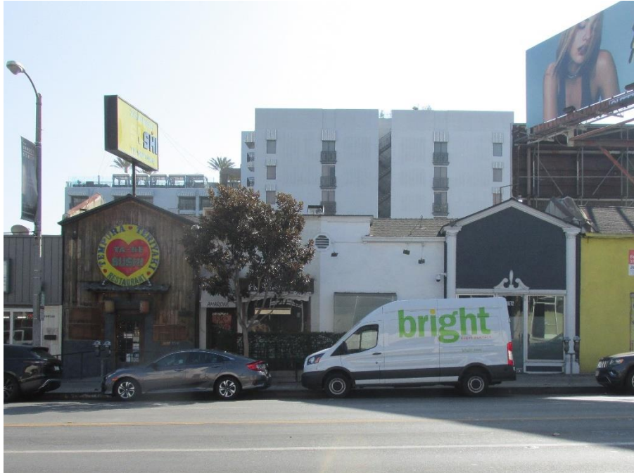
Figure 23. 8866-8872 Sunset Boulevard North Elevation, View looking south (IMG_8995)
