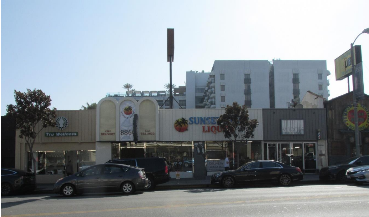
Figure 18. Building 2, 8860-8860a Sunset Boulevard (Tru Wellness, Sunset Strip Liquor, and Barcode Barber Shop), North Elevation, View looking south (IMG_8983)
