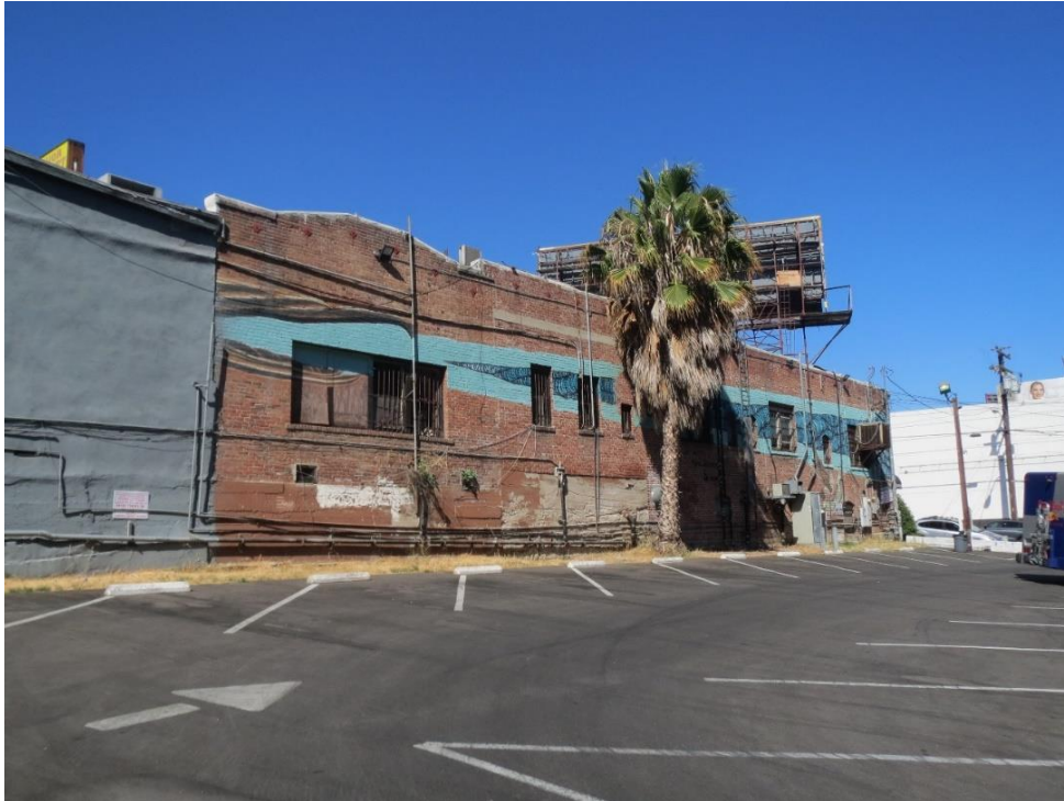
Figure 17. South elevation, View looking northeast (IMG_4105)
