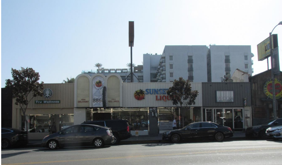
Figure 1. Building 2, 8860-8860a Sunset Boulevard (Tru Wellness, Sunset Strip Liquor, and Barcode Barber Shop), North Elevation, View looking south (IMG_8983)
