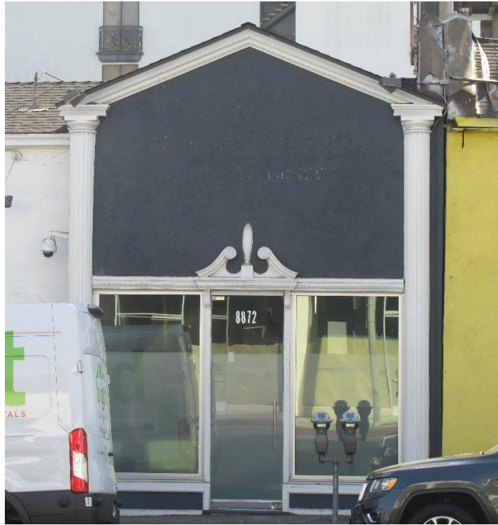
Figure 5. 8872 Sunset Boulevard North Elevation, View looking south (IMG_8998)
