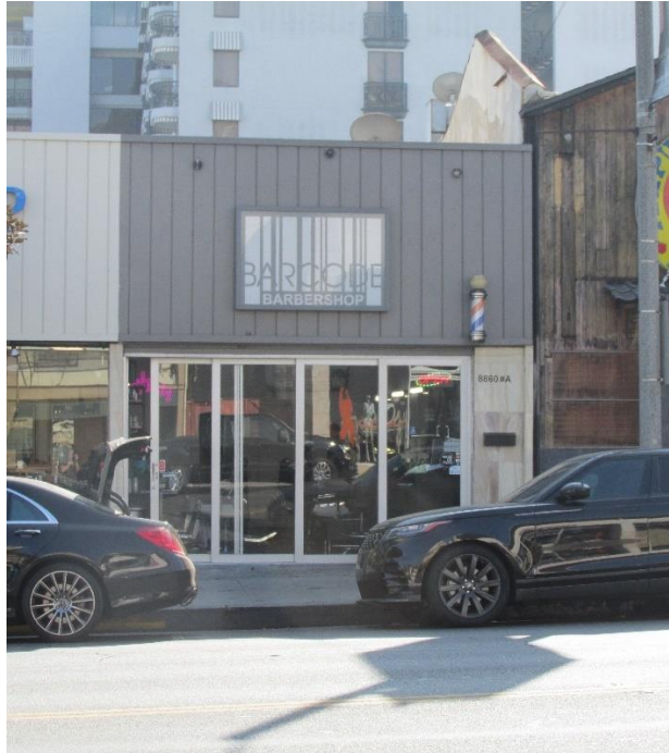
Figure 22. Storefront 3, 8860A Sunset Boulevard (Barcode Barber Shop) North Elevation, View looking south (IMG_8985)
