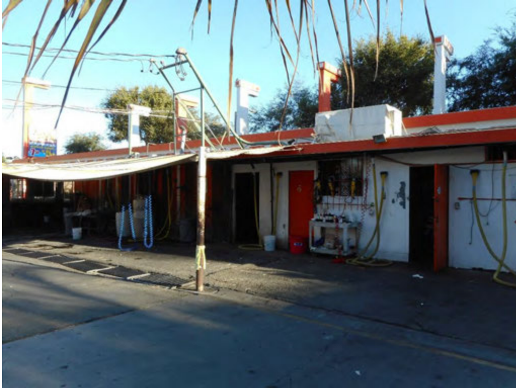
19. East end of north elevation of car wash building
