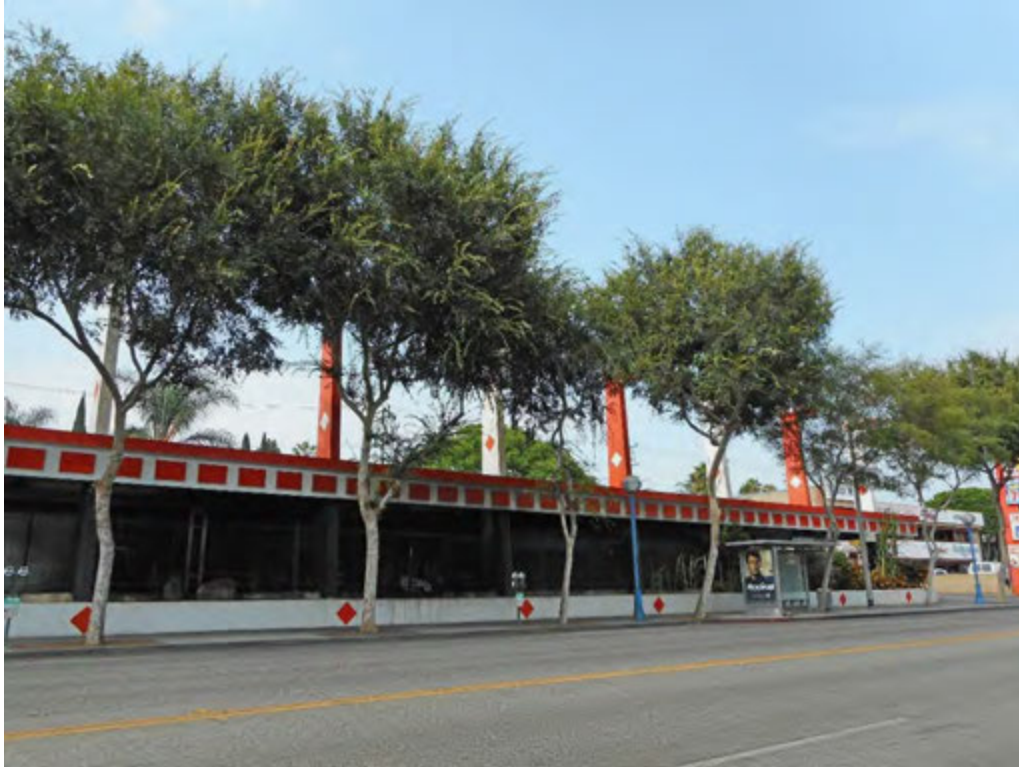
3. Middle section and east end of car wash along Santa Monica Boulevard
