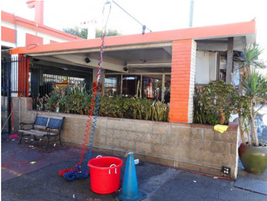
17. East elevation of waiting area attached to the north of the car wash building
