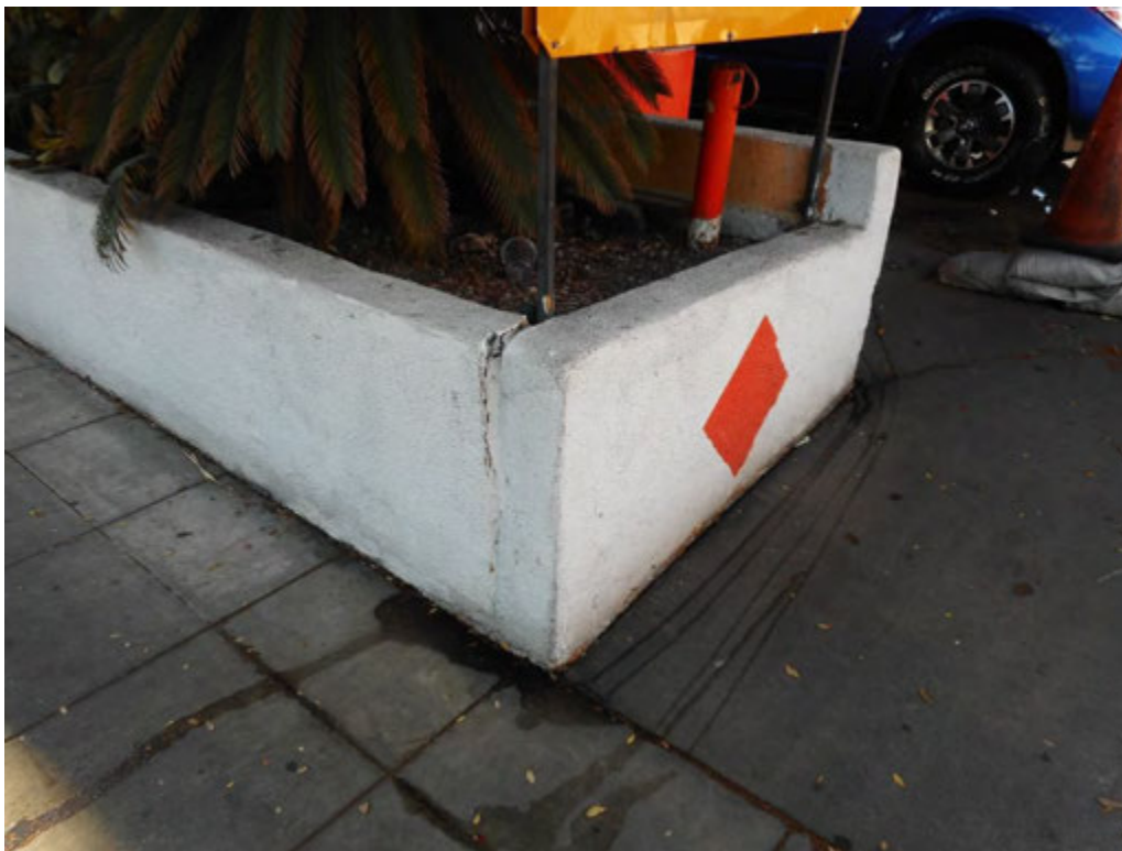
26. Detail of wall corner of car wash at Santa Monica Boulevard
