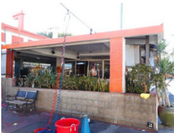
Waiting area at northeast corner of building
