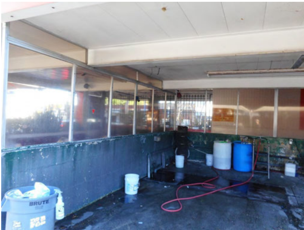
18. Car wash building interior
