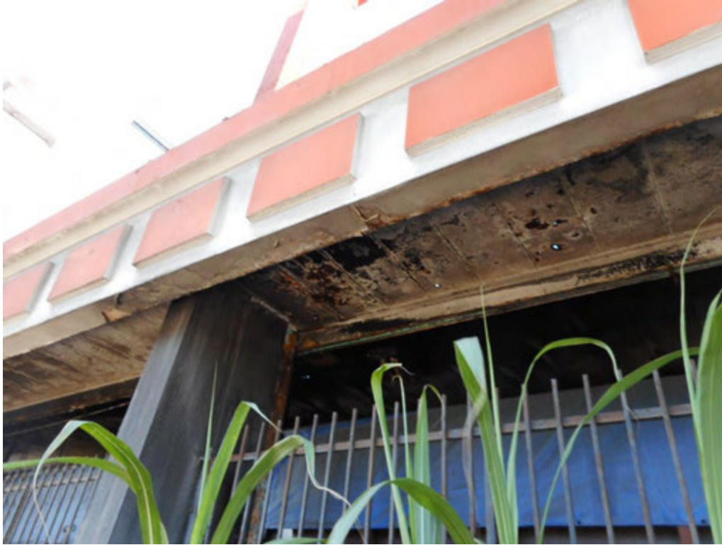
25. Detail of fascia of the car wash along Santa Monica Boulevard
