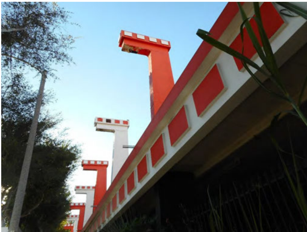
6. Upper area of south elevation along Santa Monica Boulevard
