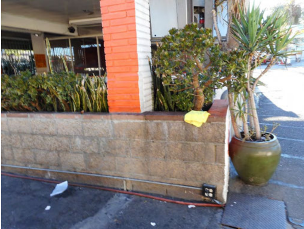
27. Detail of wall corner of car wash at northeast corner
