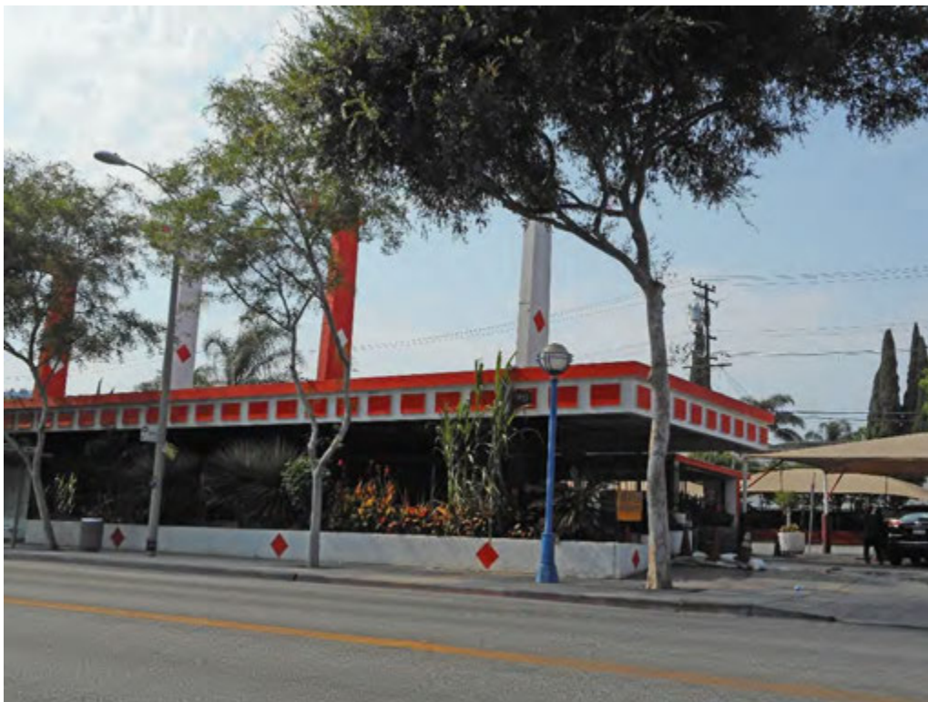
4. East end of car wash along Santa Monica Boulevard
