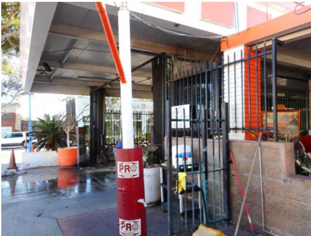
16. East elevation of car wash building
