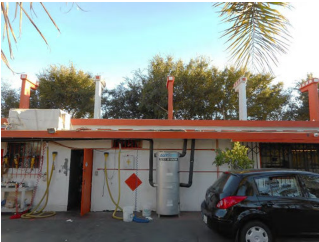
20. Middle section of north elevation of car wash building
