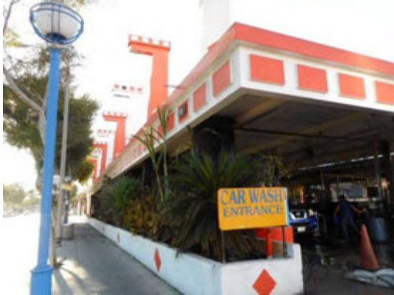
South and east elevations
