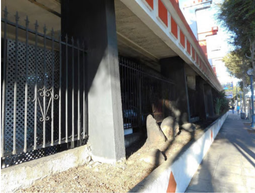
9. South elevation at street level along Santa Monica Boulevard
