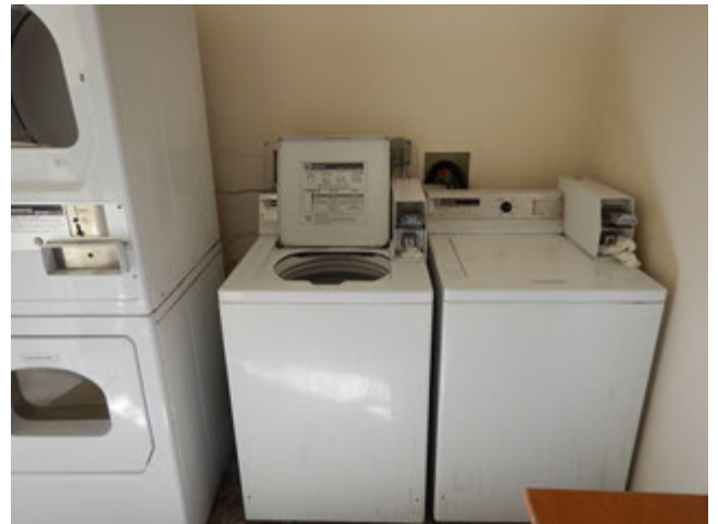
16. View of laundry room at subject property
