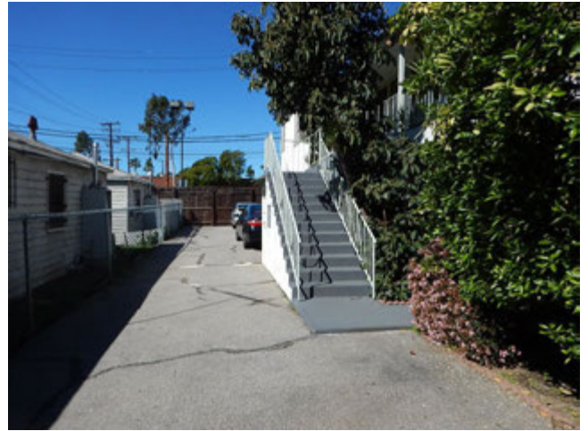
6. View of tenant access to second floor apartments at subject property
