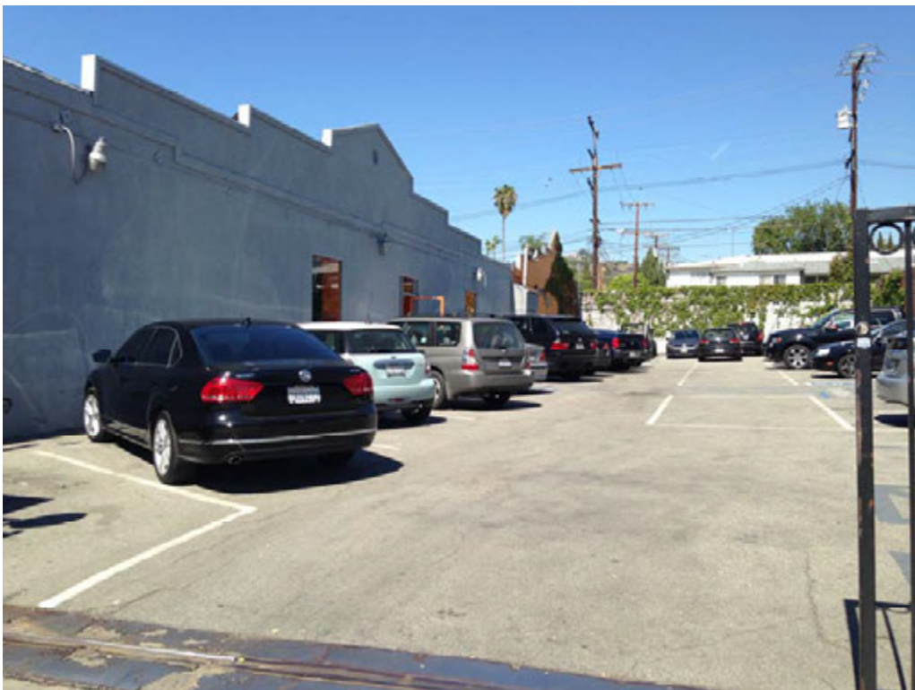
View of the parking area and east side of subject property building 7811 Santa Monica Blvd, West Hollywood
