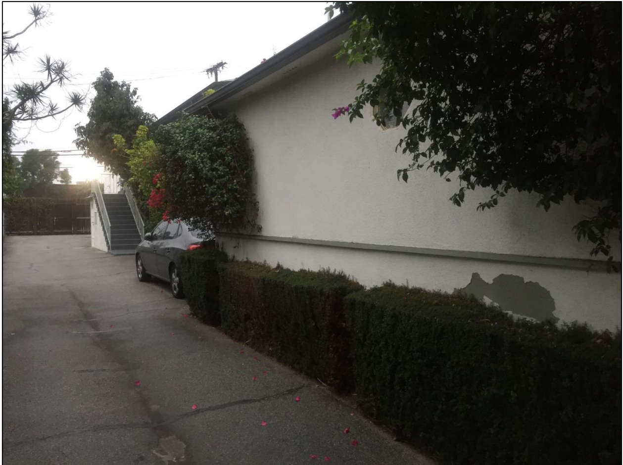
Figure 16. The south elevation of the single-family residence.
