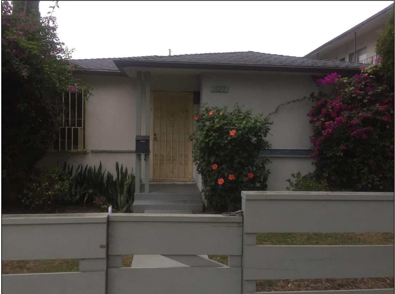
Figure 13. The east (main) elevation of the single-family residence.
