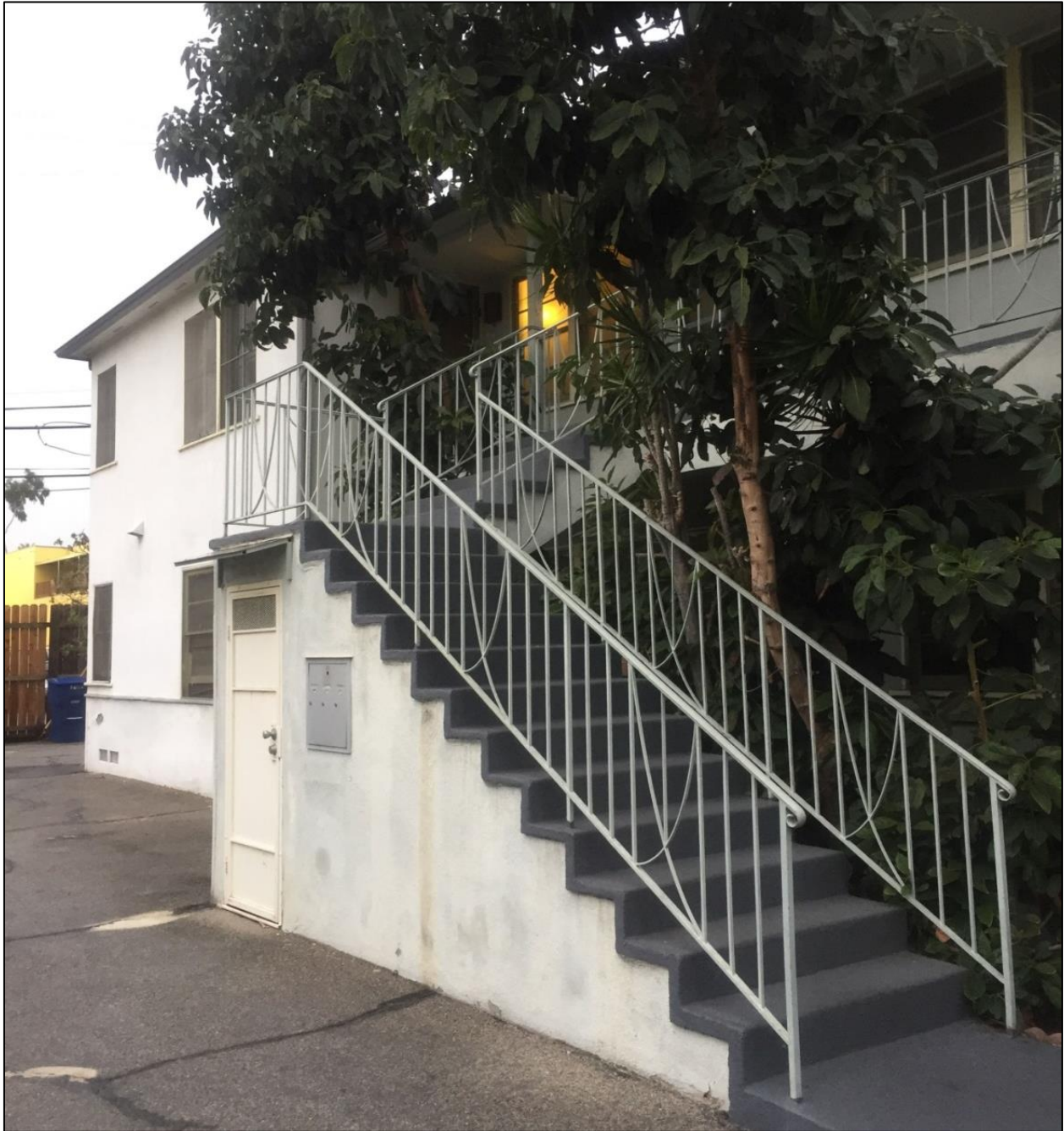
Figure 19. The west elevation of the two-story section, view looking northeast.
