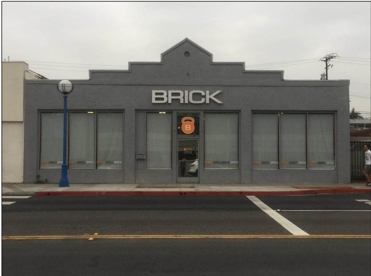
Figure 6. South (main) elevation.
