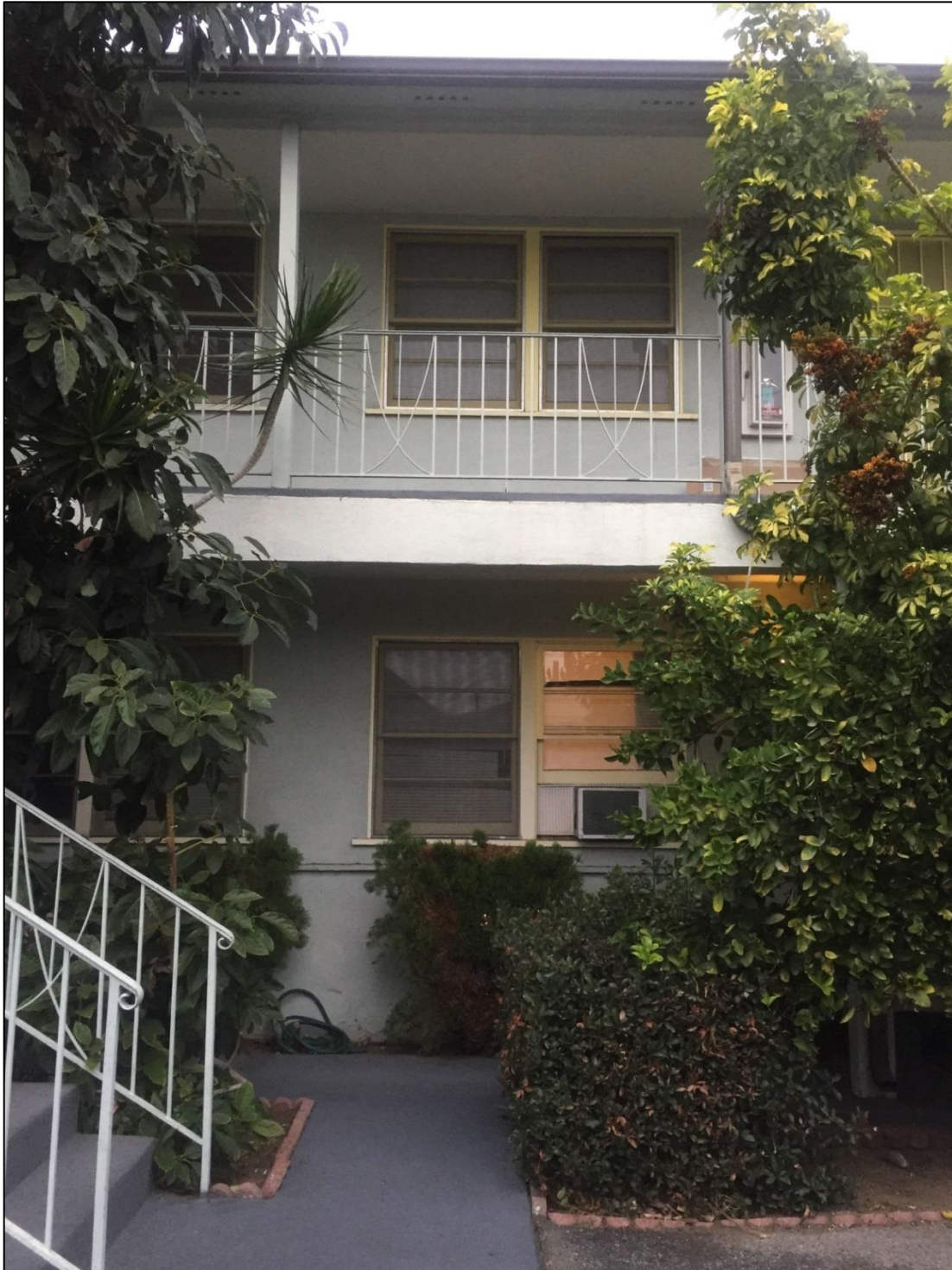
Figure 20. The west elevation of the two-story section, view looking northeast.
