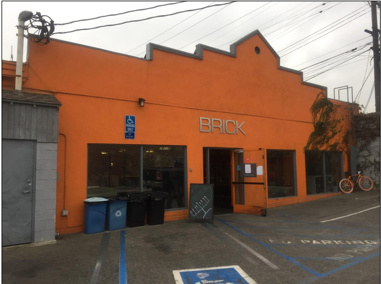
Figure 8. Detail showing the east elevation of the newer building.
