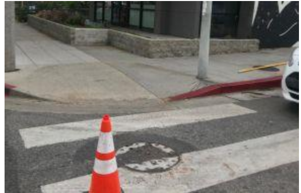
Manhole Before Install
