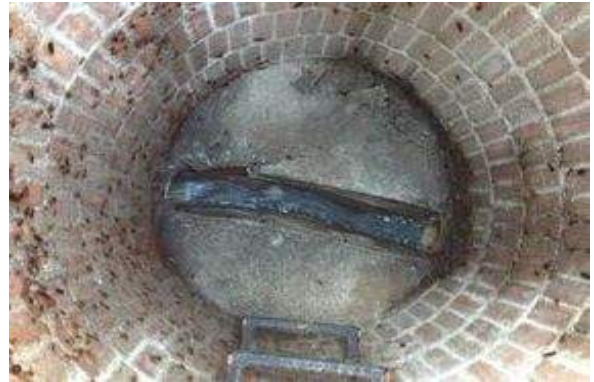
Manhole Before Install
