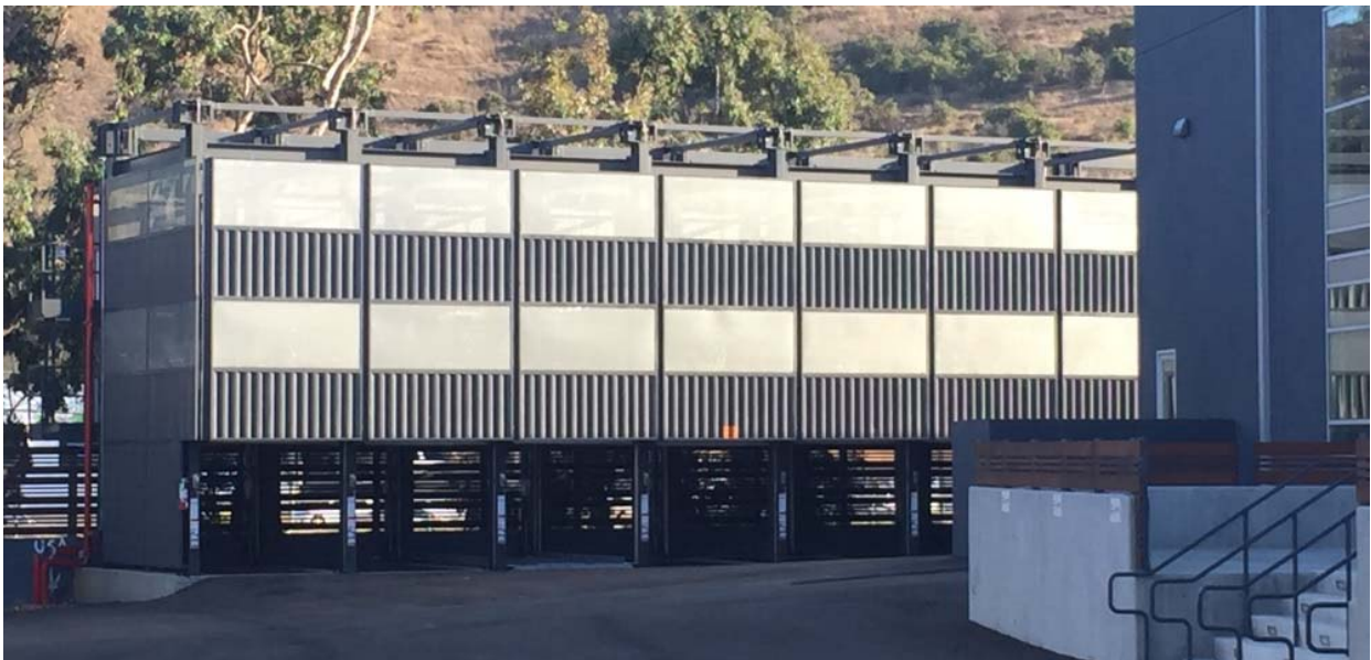
Figure 2 Example of mechanical parking on a surface parking lot with screening and covering.
