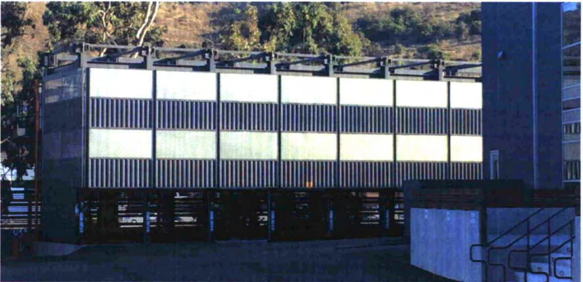
Figure 2 Example of mechanical parking on a surface parking lot with screening.
