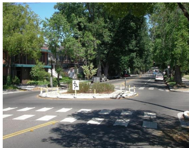
Figure 16. Example of a Traffic Circle
