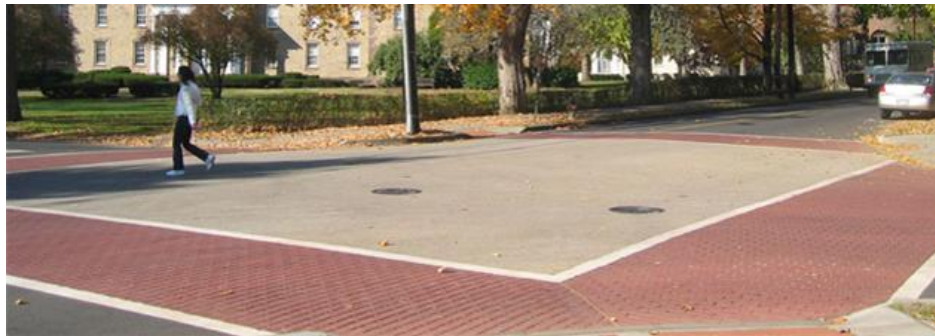
Figure 11. Example of a Raised Intersection
