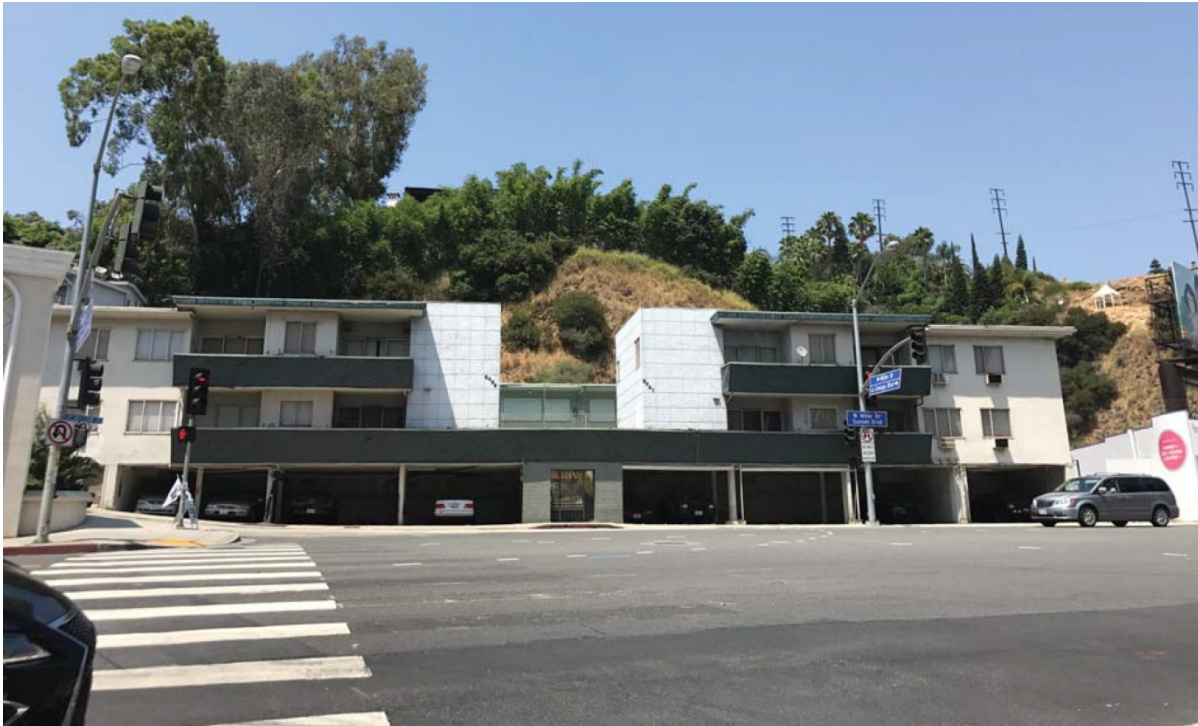
Photo 1: View of existing multi-unit residential building from Sunset Boulevard.
