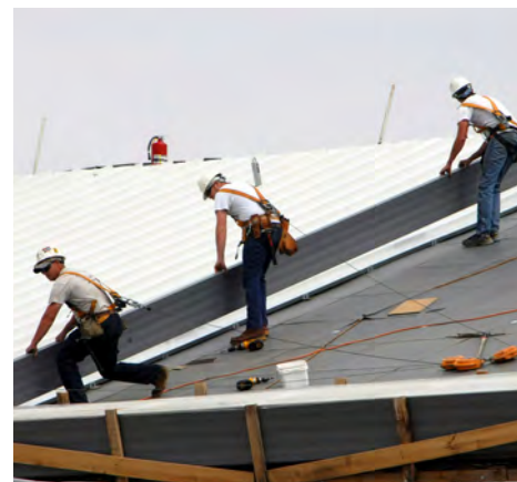
Cool roof installation
