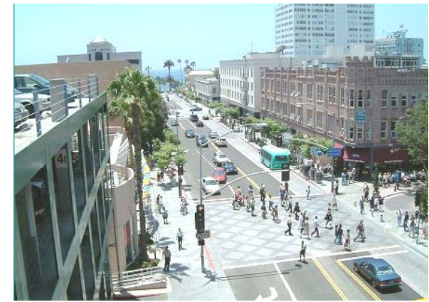
Setback stop lines and raised, painted and/or paved crosswalks improve pedestrian capacity, visibility and safety at intersections. (Photo location: Third Street Promenade in Santa Monica)
