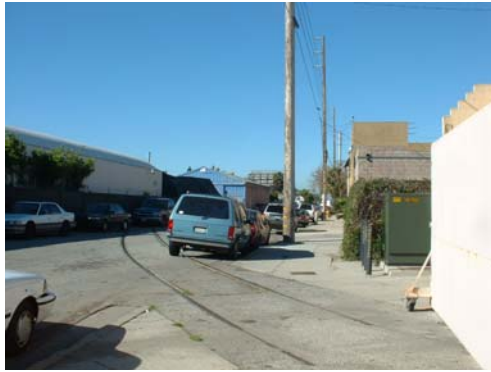
Existing industrial use and previous railroad tracks on Exposition Boulevard
