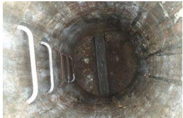
Manhole Before Install
