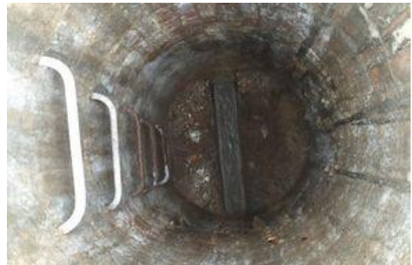
Manhole Before Install
