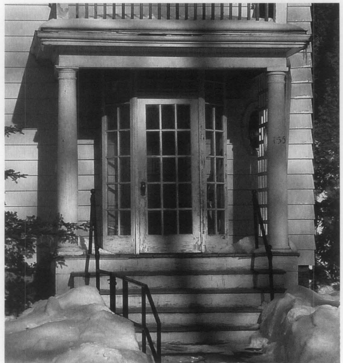
Figure 13. Particularly in New England, there is a cold weather tradition of installing temporary glass and wood panels at entrance doors, thereby creating an enclosed vestibule. These enclosures with their small divided lights were generally removed in the spring.
