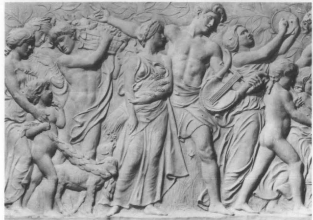
This glass fiber reinforced concrete sculptural wall panel will replace the seriously damaged resin and plaster original. A finely textured surface was achieved by spraying the GFRC mix into molds that were created from the historic panel and resculpted based on historic photographs. Photo: Courtesy of MJM Studios.
