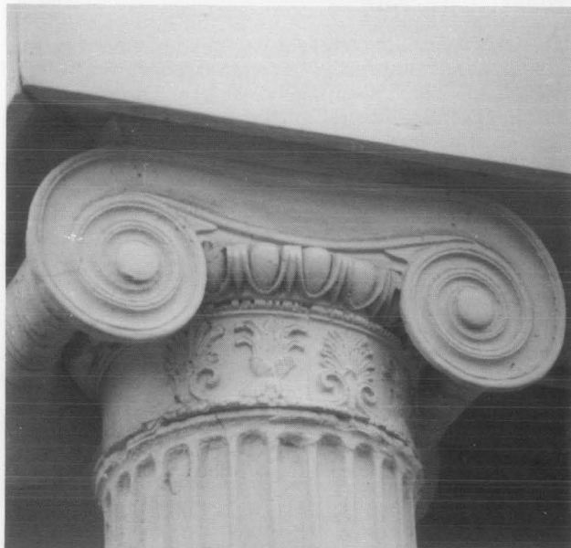
This replica column capital was made using epoxy resins poured into a mold taken from the building. The historic wooden column shaft was repaired during the restoration. Photo: Courtesy Dell Corporation.
