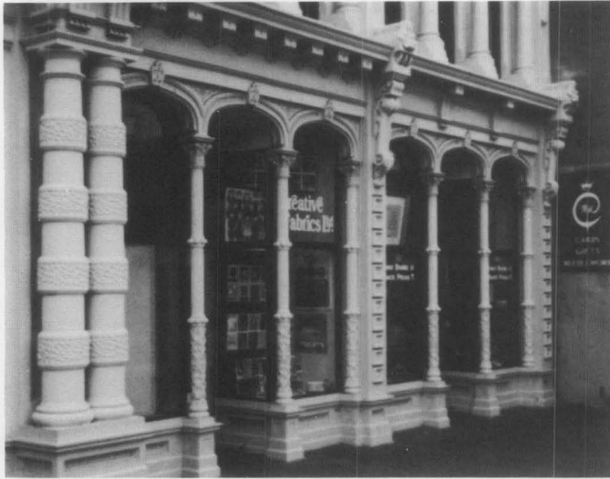
Illus. 11. The unavailability of historic craft techniques is another reason to consider substitute materials. The original first floor cast iron front of the Grand Opera House, Wilmington, DE, was missing; the expeditious reproduction in cast aluminum was possible because artisans working in this medium were available. Photo: John G. Waite.
