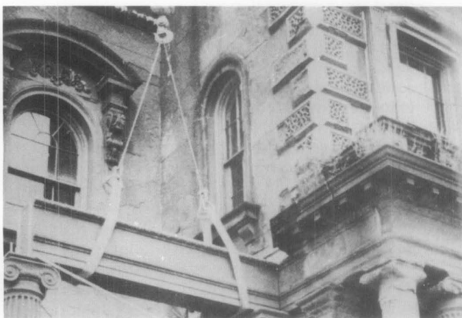
Illus. 9. Simple solutions should not be overlooked when materials are no longer available. In the case of the Morse-Libby Mansion (1859), Portland, ME, the deteriorated brownstone porch beam was replaced with a carved wooden beam painted with sand impregnated paint. Photo: Stephen Sewall.
