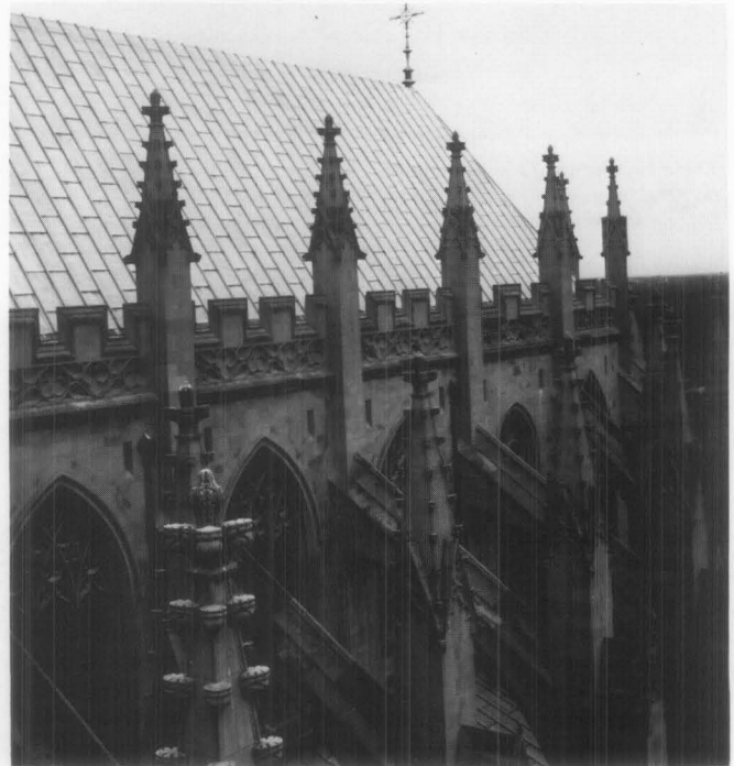
Good design and quality materials for the roof surface, fastenings, and flashing minimize roofing failures. This is essential on roofs such as on the National Cathedral where a thorough maintenance inspection and minor repairs cannot be done easily without special scaffolding. However, the success of the roof on any structure depends on frequent cleaning and repair of the gutter system. (Washington, D.C., photo courtesy of John Burns, A.I.A.)
