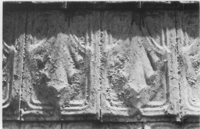
Tin shingles, commonly embossed to imitate wood or tile, or with a decorative design, were popular as an inexpensive, textured roofing material. These shingles 8\frac{3}{8} inch by 12\frac{1}{2} inch on the exposed surface) were designed with interlocking edges, but they have been repaired by surface nailing, which may cause future leakage. (Ballard House, Yorktown, Virginia, photo by Gordie Whittington, National Park Service)
