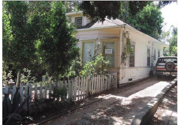
Front view of 927 N. Palm Avenue, facing southwest on N. Palm Avenue.
