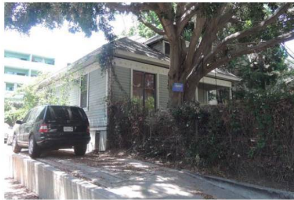
Front view of 931 N. Palm Avenue, facing northwest on N. Palm Avenue.
