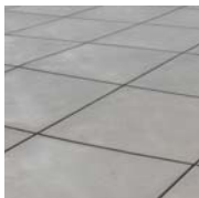
B Concrete paving with integral color
