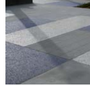
C Scored and colored concrete paving
