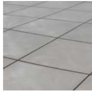
B Concrete paving with integral color
