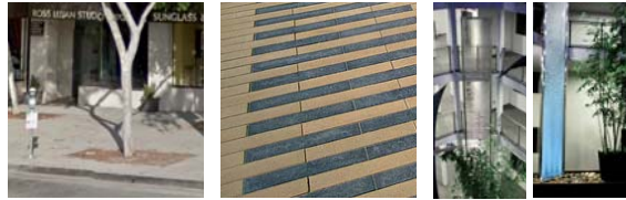
A Scored conc. paving to match existing sidewalk specifications B Linear conc. paving to enhance and differentiate entrances C Water veil fountain 20' - 30' h with changing LED lights
