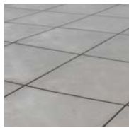
B Concrete paving with integral color
