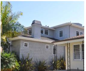
☑ This second-story addition is integrated into the original design through the modulation of its components and forms.
