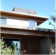
Mechanical screen integrated with building design.
