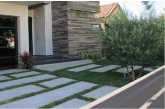
☑ Light-colored paving that is integrated with planting reduces stormwater run-off and urban heat island effect.
