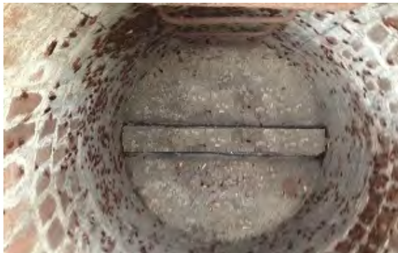
Manhole Before Install
