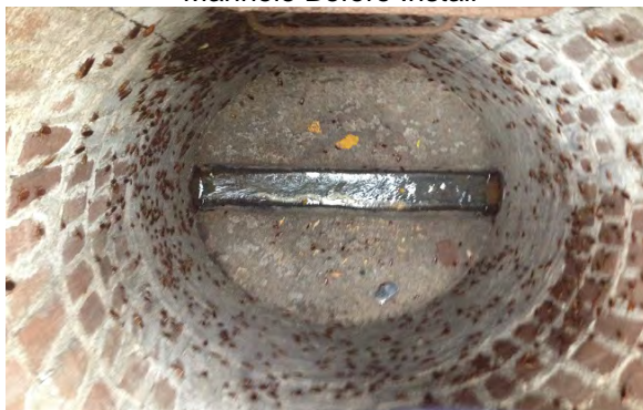
Manhole Before Install
