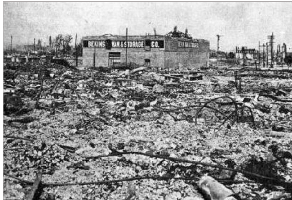
Figure 15. An image of the sole surviving Bekins Van & Storage, Co. in San Francisco, CA, which had been constructed using Kahn's Trussed Bar (Trussed Concrete Steel Company Brochure, 1906).
