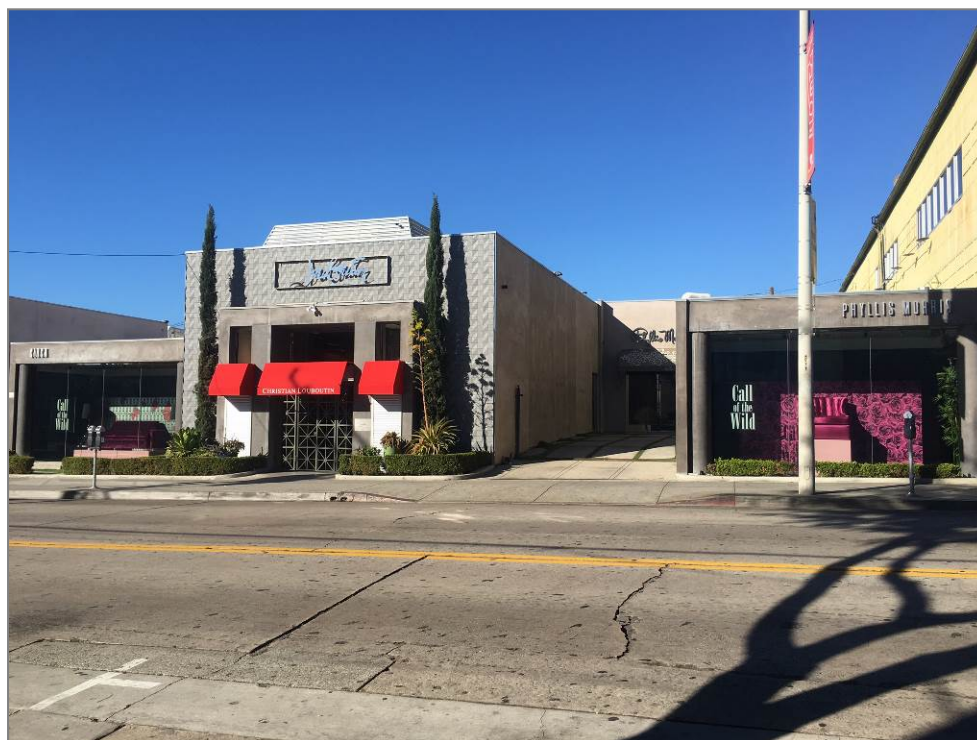
Figure 3. 655-657 N. Robertson Blvd., east and north elevations, view southwest (ARG, 2016).
