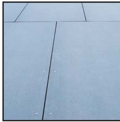
9 FIBER CEMENT CLADDING
