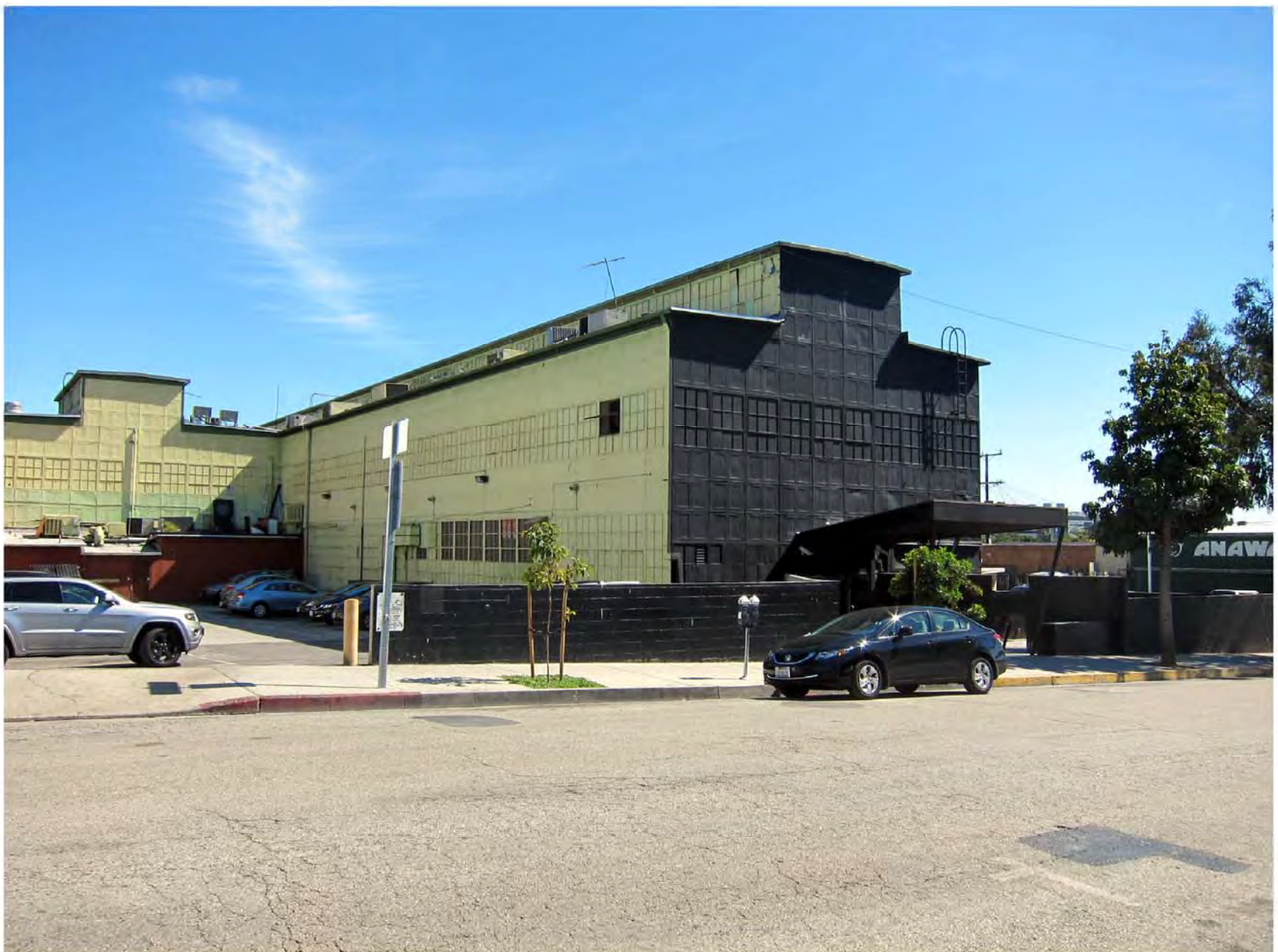
Photo 2: View southeast from North La Peer Avenue across project site towards surface parking lot and the Factory building
