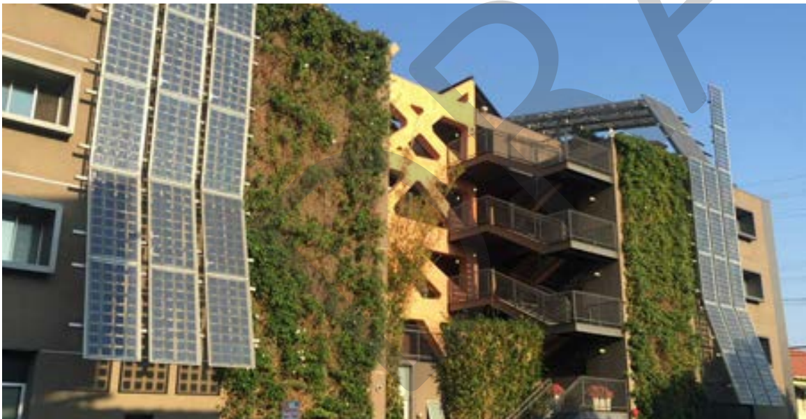
Buildings like the Sierra Bonita Apartments have reduced utility costs for tenants by installing solar arrays on the roof and side wall of the building.
