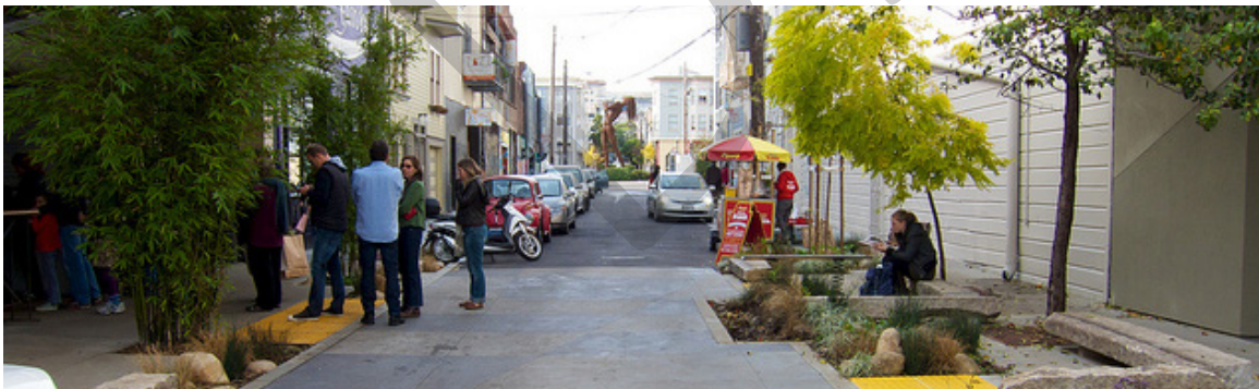
A major transformation of Linden Alley in San Francisco, CA, includes bioswales, new paving, and seating areas.
