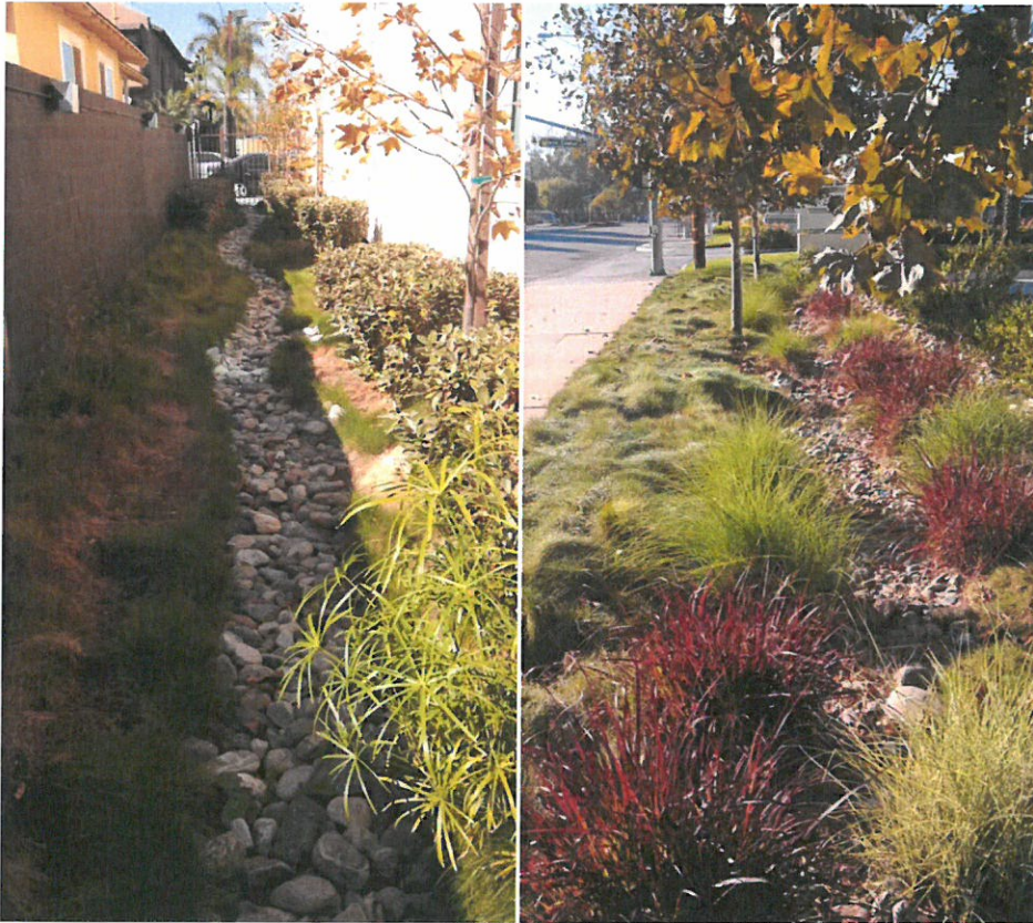
Figure 2: Vegetated Swale (Seal Beach, CA).
