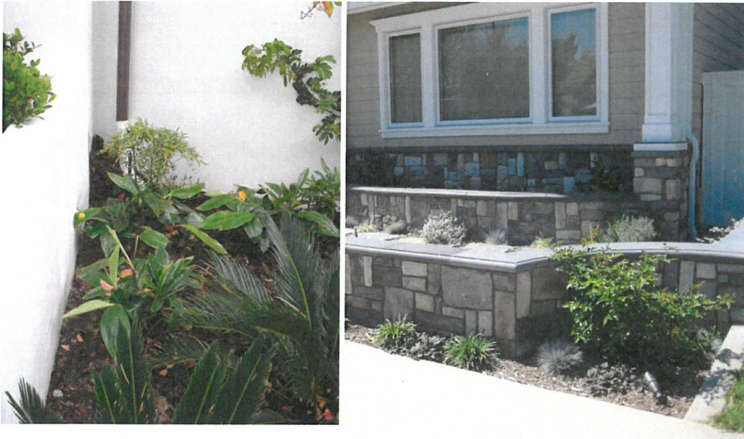
Figure 1: Flow-through planter box (Seal Beach, CA – Left; Rancho Palos Verdes, CA – Right)
