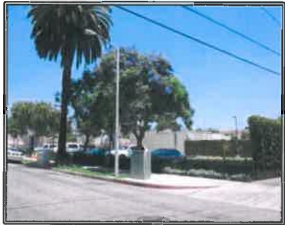
A view of the subject looking northeast from Spaulding Avenue.
