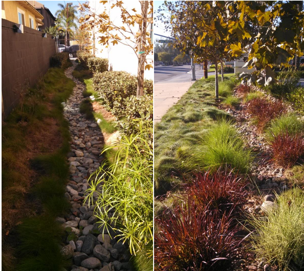
Figure 2: Vegetated Swale (Seal Beach, CA).
