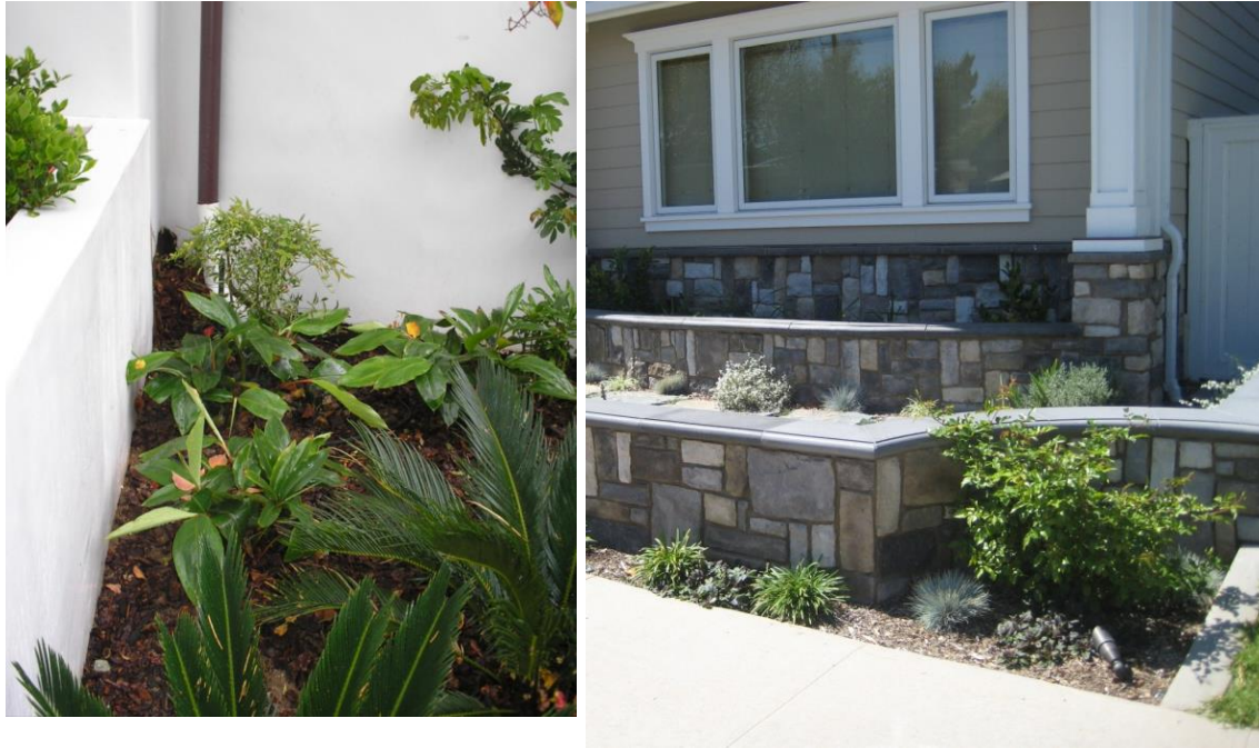
Figure 1: Flow-through planter box (Seal Beach, CA – Left; Rancho Palos Verdes, CA – Right)
