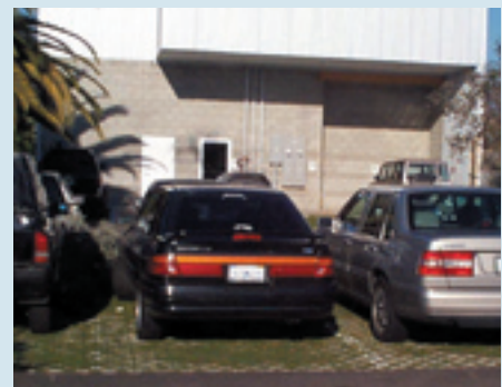
<Parking lot of small office building made of concrete permeable pavers>
