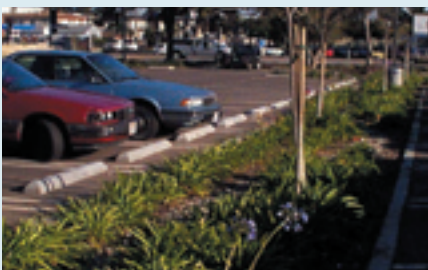
<Institutional parking lot biofilter>
