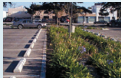
<Parking lot runoff enters biofilter for treatment and percolation>
