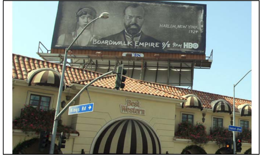
Photo 2: 8400 Sunset Boulevard Roof Mounted
