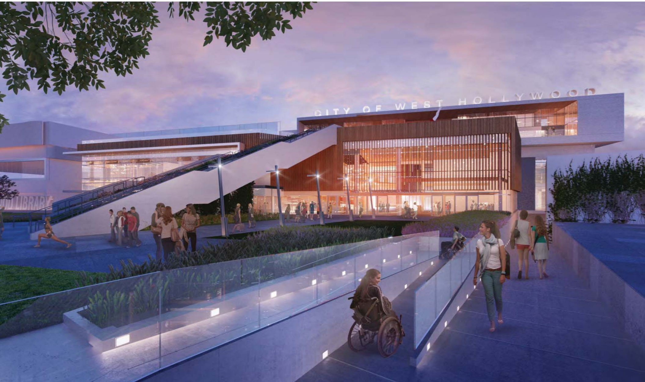
VIEW TOWARD ENTRY
