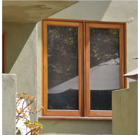
☑ Quality wood window with simple detailing.
