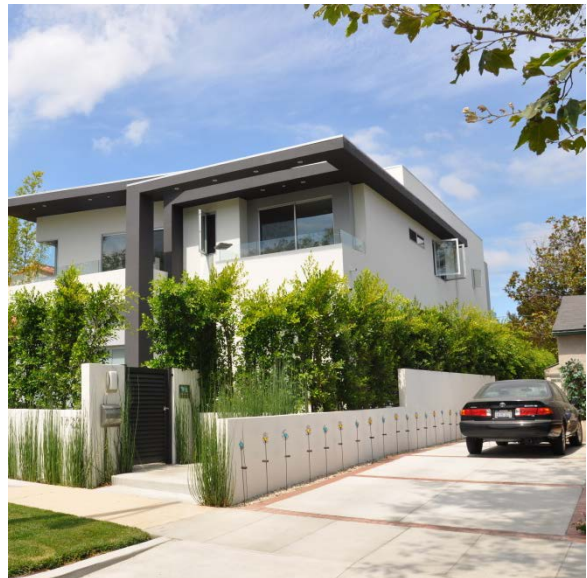
⊘ The two-story side wall of this new development looms over its bungalow neighbor.
