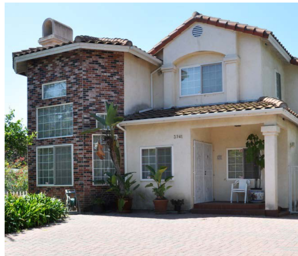
⊗ The transition between brick and stucco is poorly conceived, creating an unintegrated and unfinished appearance.
