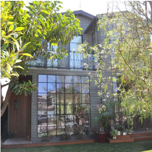
⊗ The window proportions are over-scaled and do not integrate with the traditional residential façade forms.
