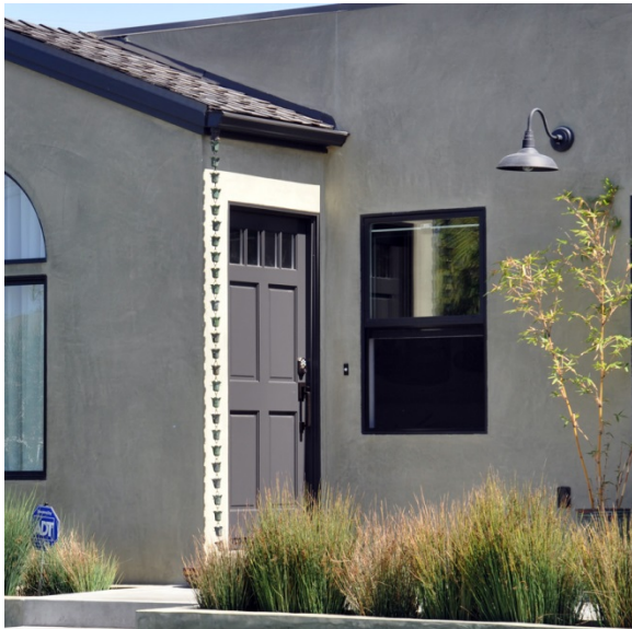
☑ “Rainchains” add visual interest to an ordinary gutter and downspout system.
