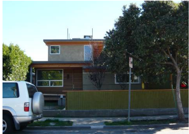
☑ This second-story addition is set back from the ground floor to reduce apparent size.
