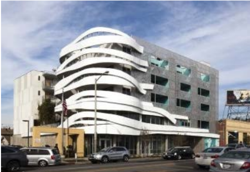
Courtyard at La Brea Affordable Hsg (2014)
