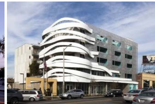
Courtyard at La Brea Affordable Hsg (2014)
