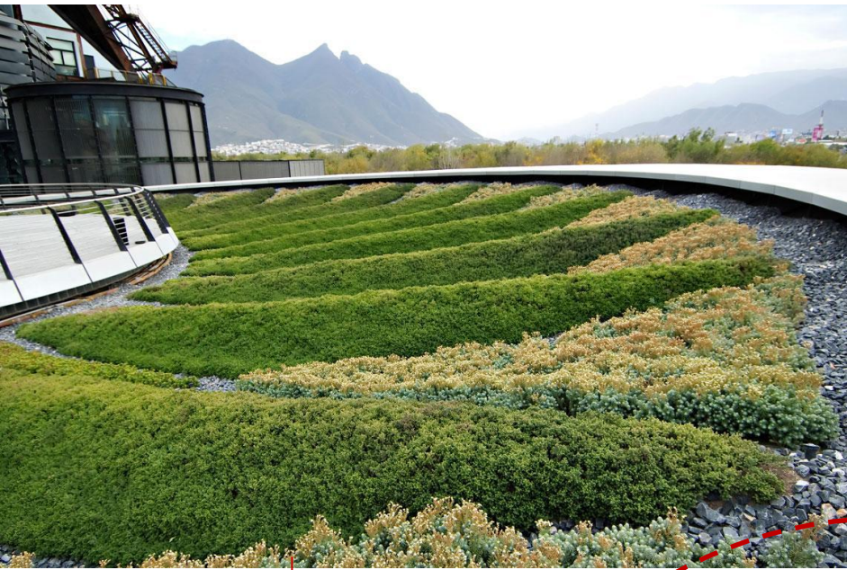
Green Roof Planting
