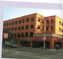
Example of park once garage with pedestrian-friendly ground floor retail, awnings and shading devices, landscaping, window openings, driveways relegated versus primary pedestrian street.
