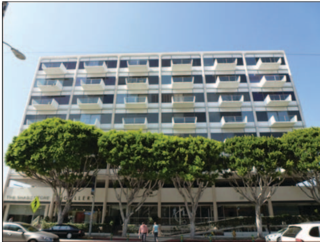
View 3: South elevation of the Existing Building looking north.
