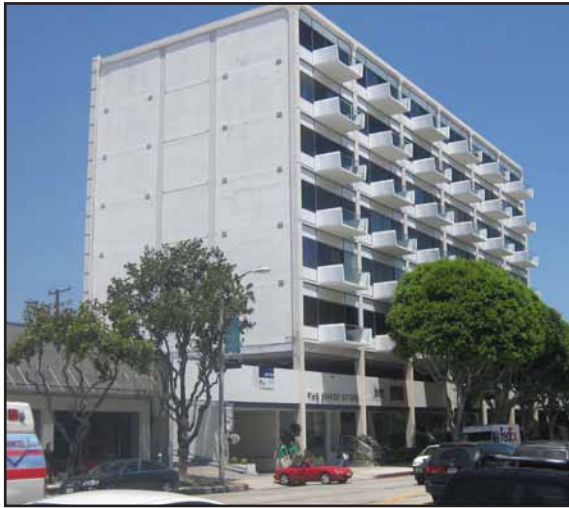
View 1: View of Existing Building across Beverly Boulevard looking northeast.
