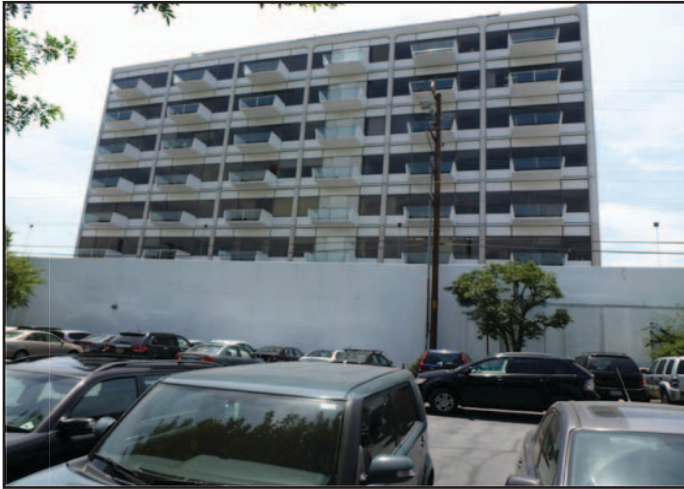
View 5: North elevation of the Project Site looking south.
