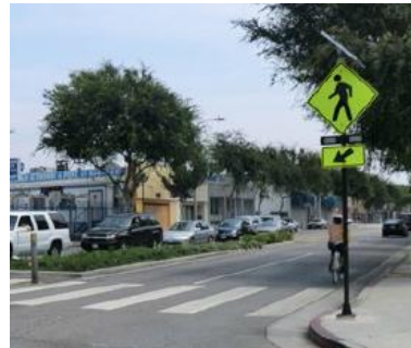
Rapid Flashing Beacon
