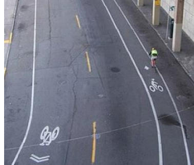
Uphill Bike Lane / Downhill Sharrow
