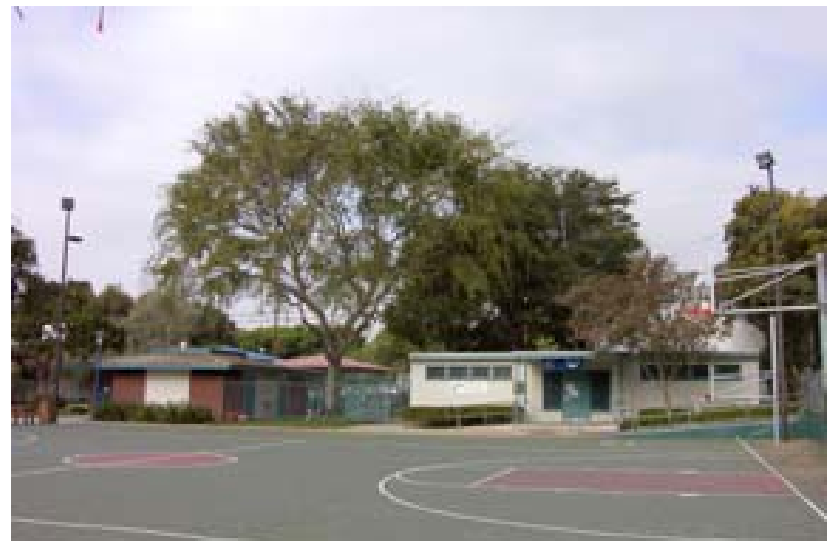
Basketball Courts divide the 'heart of the park' from the ballfield. The asphalt paving is a large impermeable area that lacks seating and shade.
