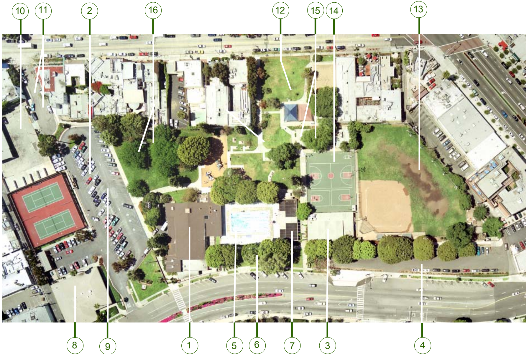
The Existing Park. Buildings, outdoor recreation facilities, fences and walls crowd the 6.6 acres of the park to the extent that realistically only 1 acre is left for what most would consider legitimate park open space.
