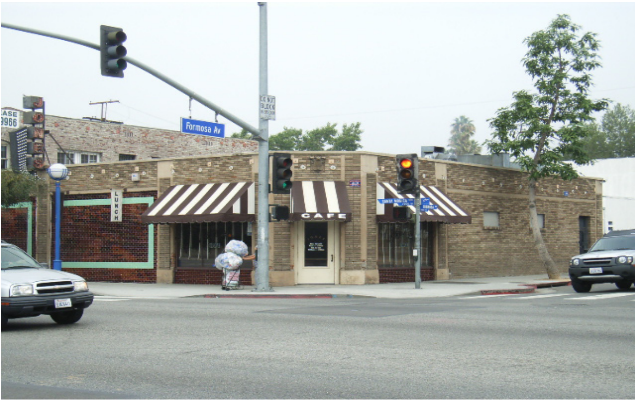
Figure 3.1-9 View across Santa Monica Boulevard toward the cafe at the corner of Formosa Avenue
