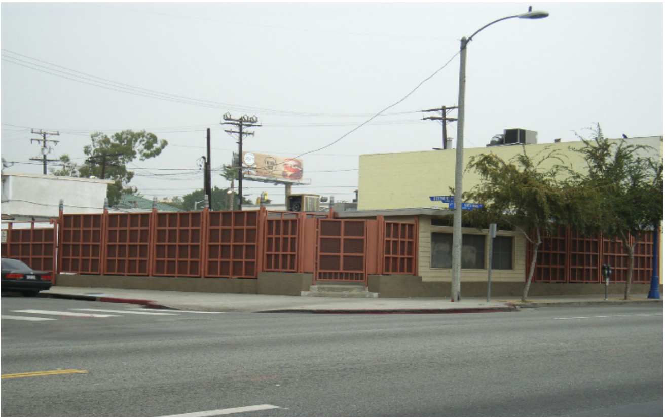
Figure 3.1-10 Parking lot and buildings on the corner of Santa Monica Boulevard and Detroit Avenue
