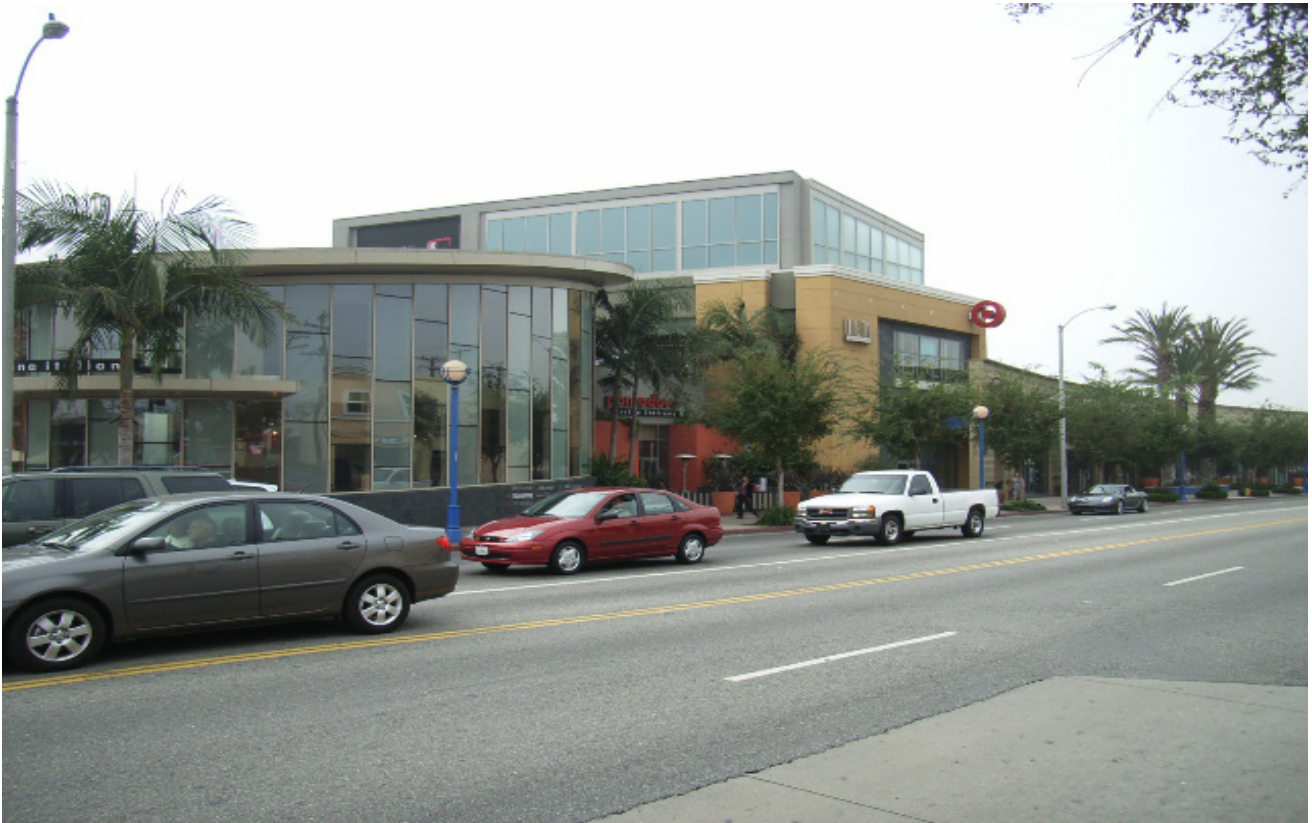
Figure 3.1-5 View southwest toward the Retail Complex on the south side of Santa Monica Boulevard
