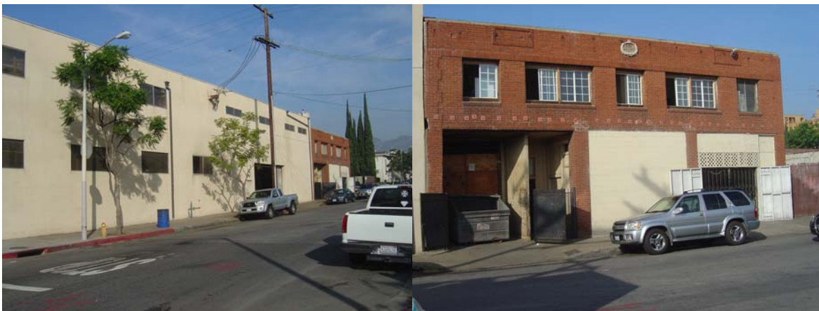
Plate 3. Façade of Buildings 2-5 along Detroit Street, with Detail of Building 2 on the right
